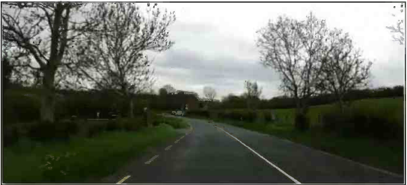
Typical non-improved rural section of R178
