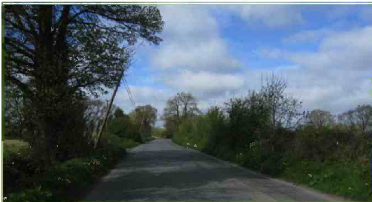
Typical rural section of the L1002
