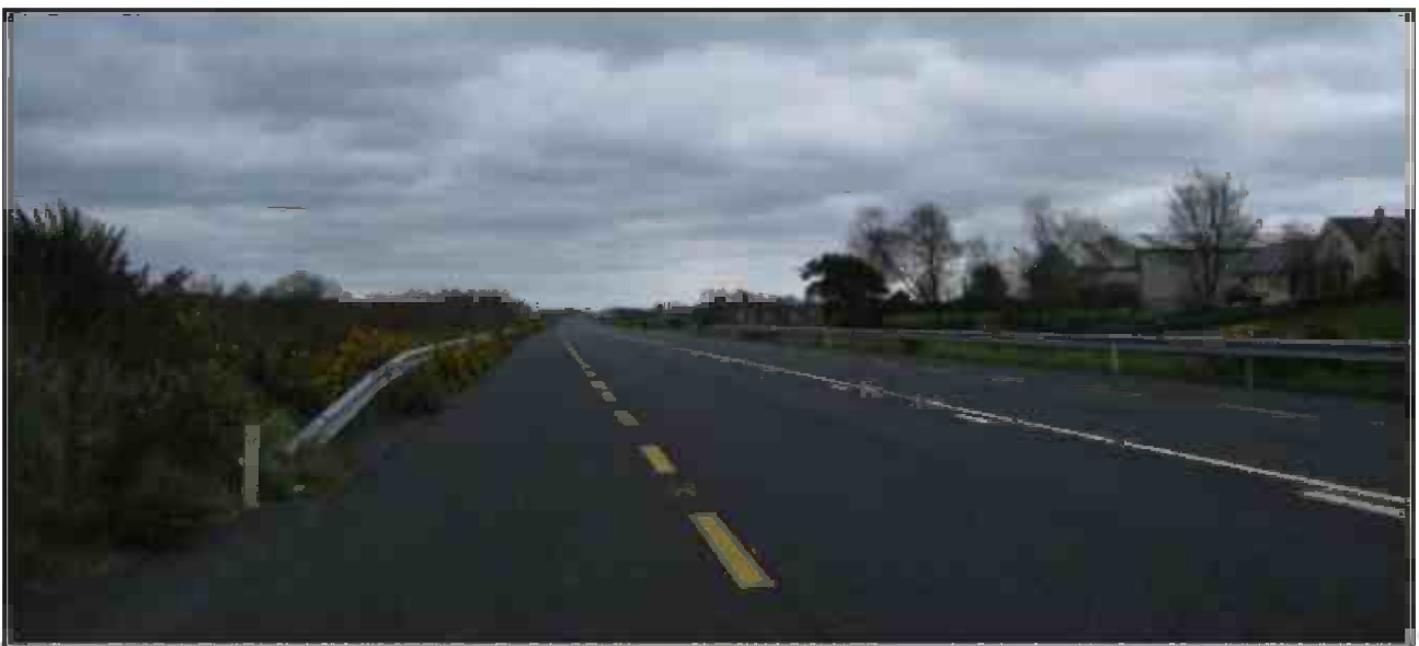
Improved rural section of R178 between Essexford and Rosslough.
