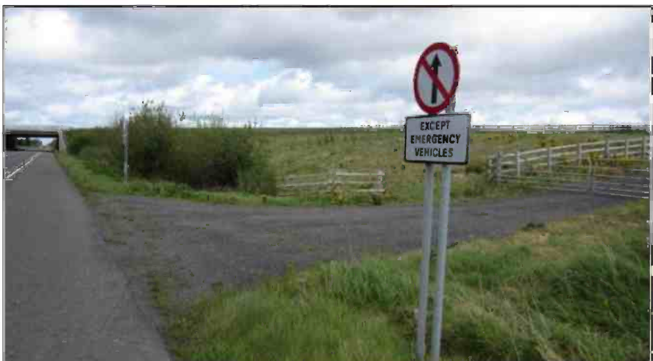
Looking along the R445 towards the M7 overbridge
