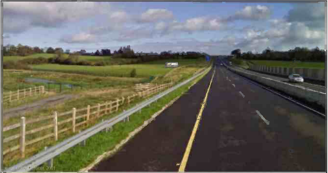
Existing access road and attenuation pond from M7 eastbound.
