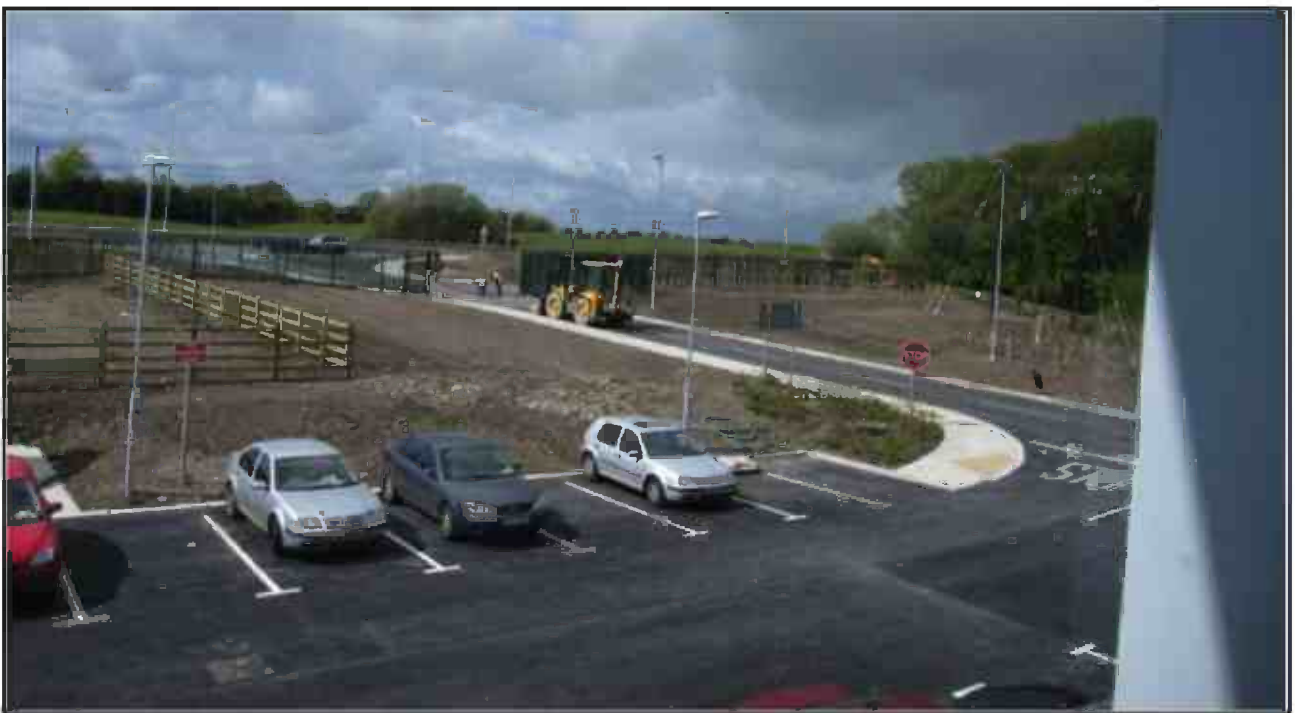
Possible site on right side of entrance to maintenance depot.
