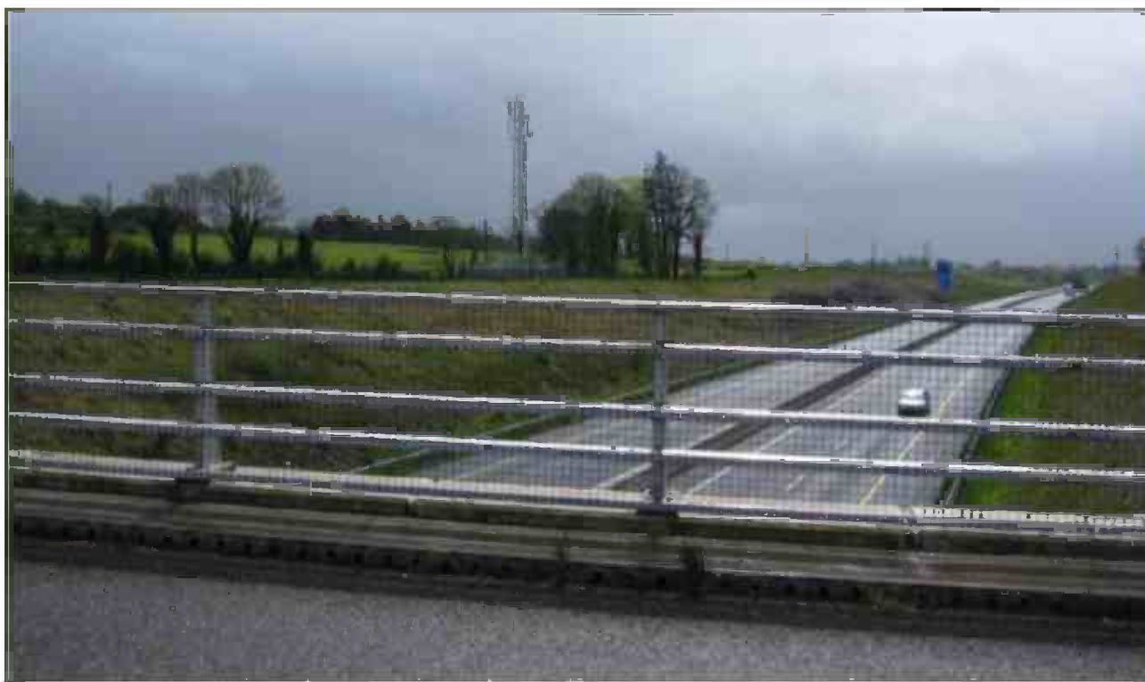
Existing mast from overbridge at Ballynahinch.
