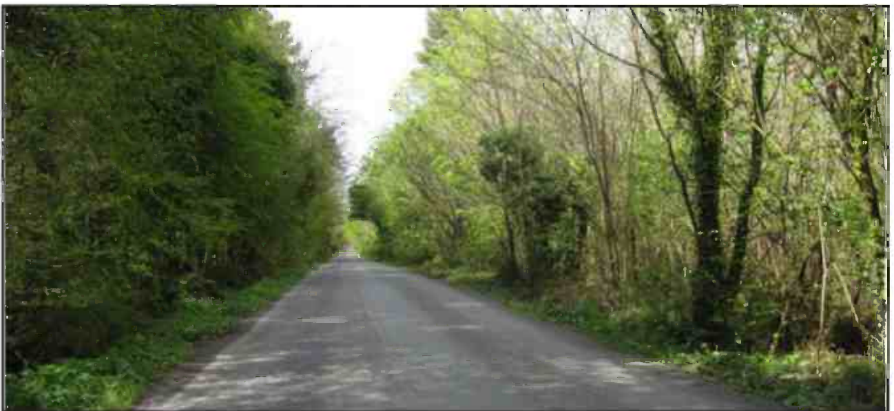
Typical rural section of the L2007
