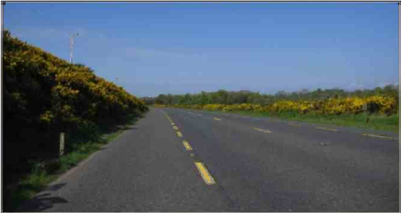
Improved rural section of N30 between Jamestown and Moneytucker.
