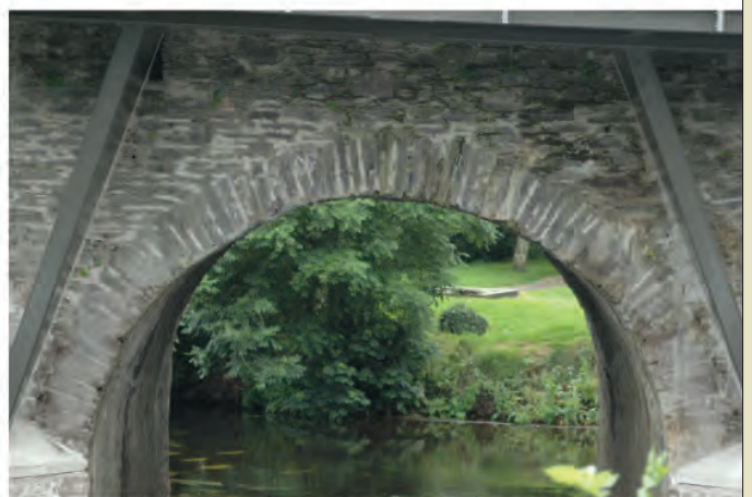
Sample of semicircular arches on Macroom Bridge: (top) south-facing arch on original late 17th-century bridge, (middle) south-facing blocked arch at the western end, corresponding to Arch 10, and (bottom) arch on northern extension of bridge. (Image: Ken Hanley)
