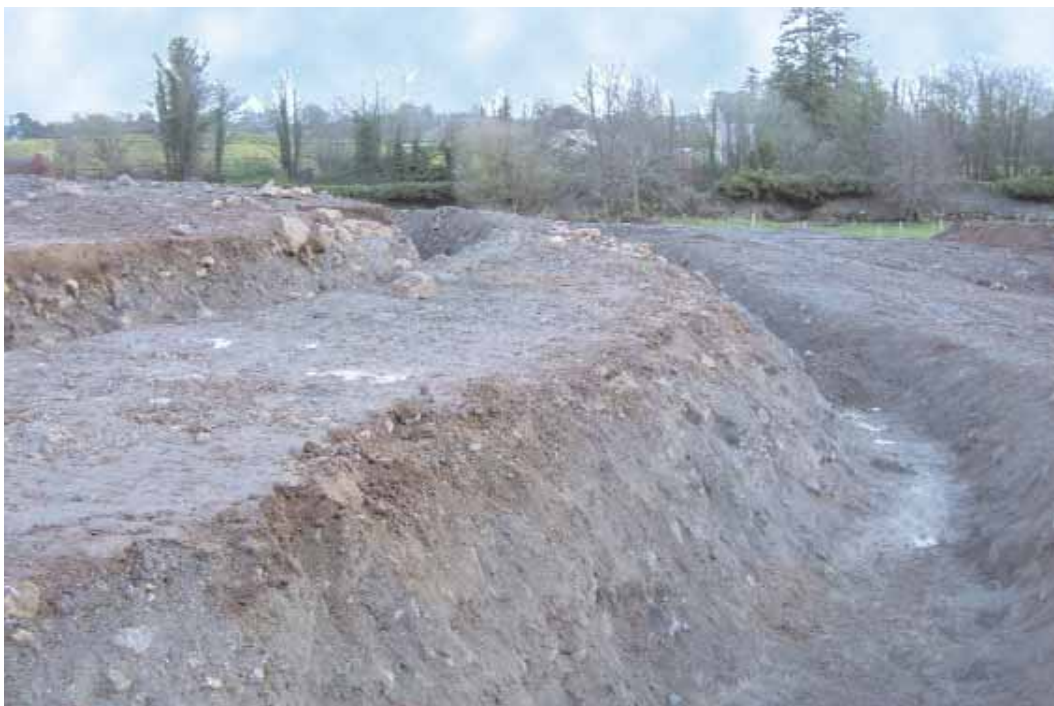
Illus. 5—The southern sections of the inner and outer ditches, looking south-east (Valerie J Keeley Ltd)
