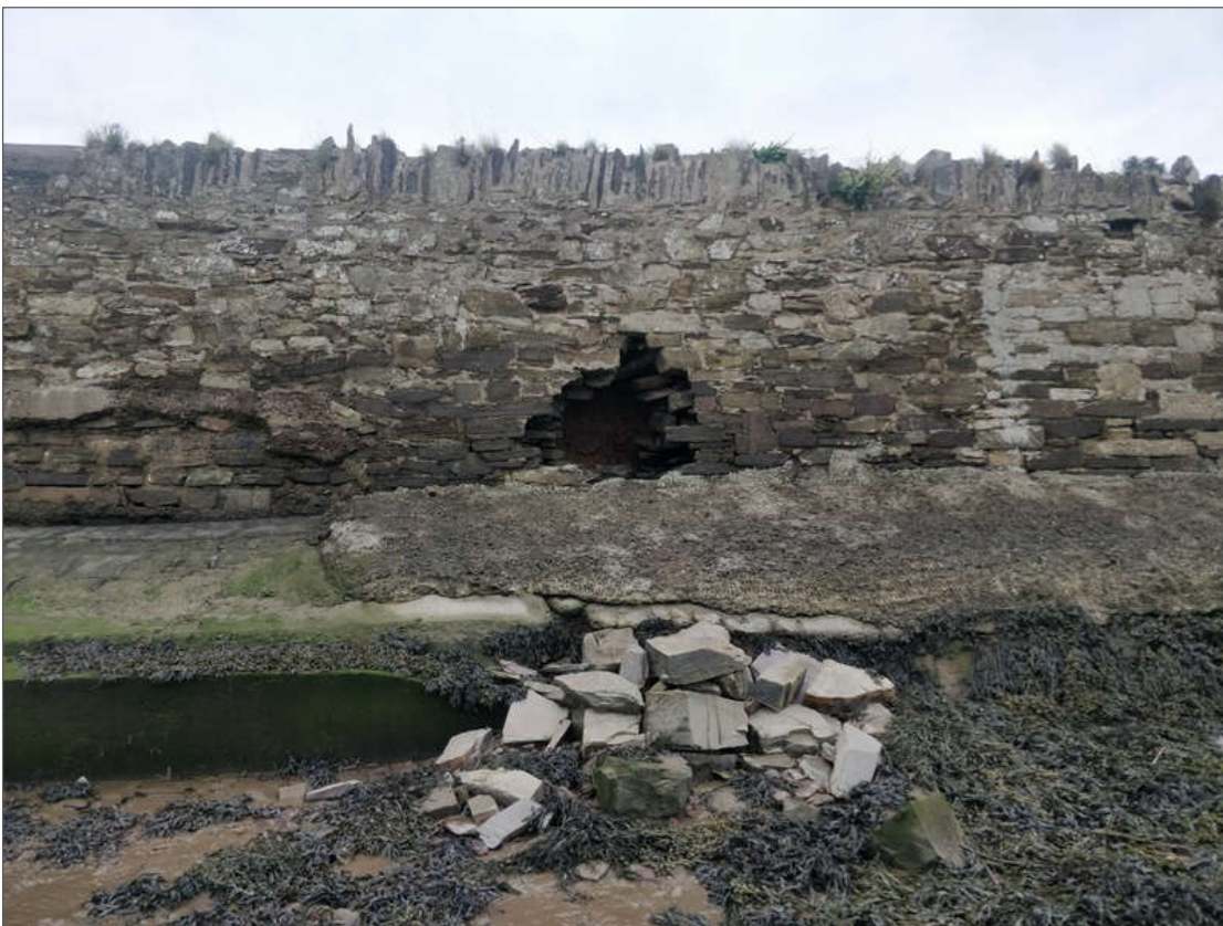
Plate 3-3 – Larger section of retaining wall to be repaired.
