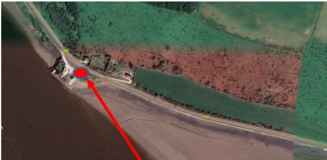
Site Compound Location
