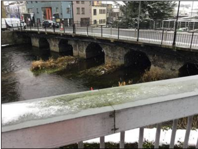
Plate 1.1 River Suir Bridge.
