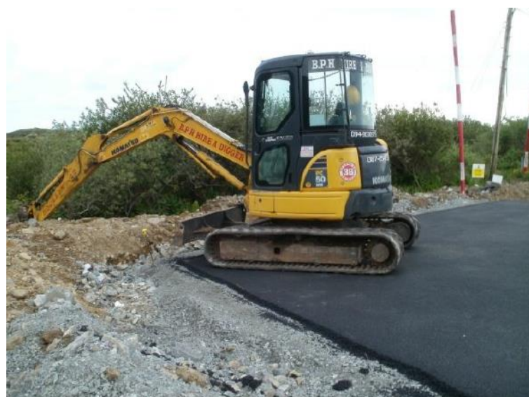
Figure C.3 Lightweight backacter for cycleway construction
