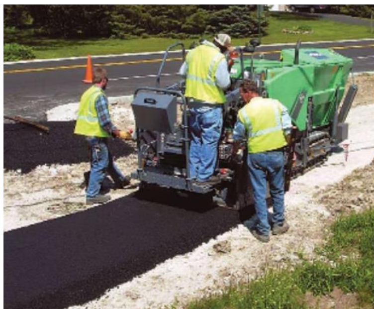
Figure C.1 Narrow width bituminous material paver
