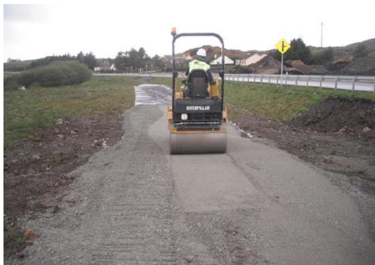
Figure C.2 Lightweight roller compactor equipment for cycleway construction
