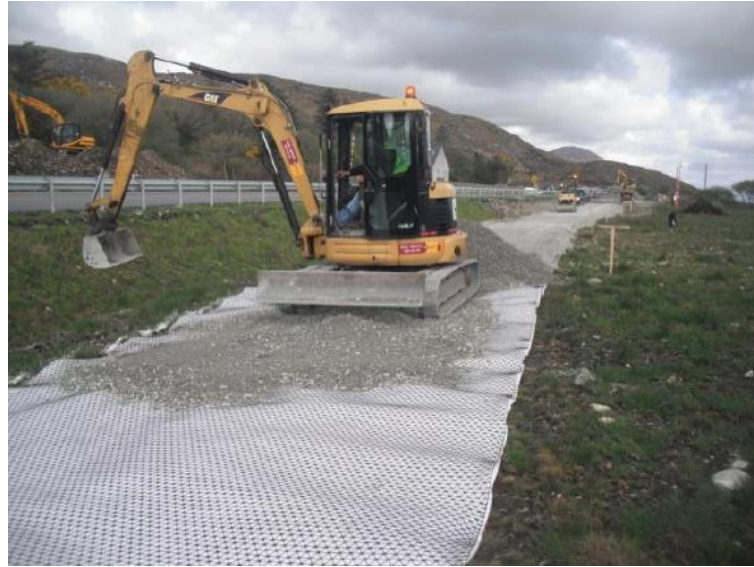
Figure C.4 Geotextile reinforced unbound granular layer construction
