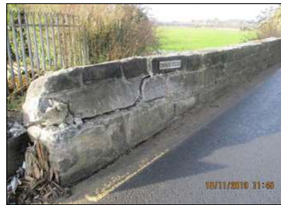
Plate 1. Downstream of Killydoon bridge with damaged parapet to the right.
