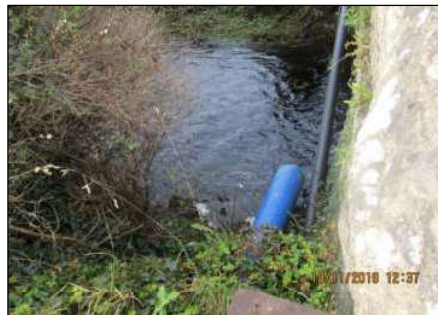
Plate 2. Discharge pipe downstream of the bridge. [Source: Atkins R.E.; 18/11/2019]
