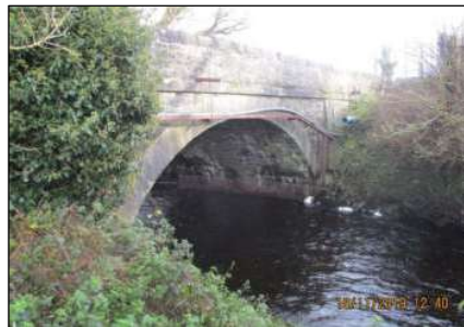
Plate 1. Downstream of Killydoon bridge with damaged parapet to the right.
