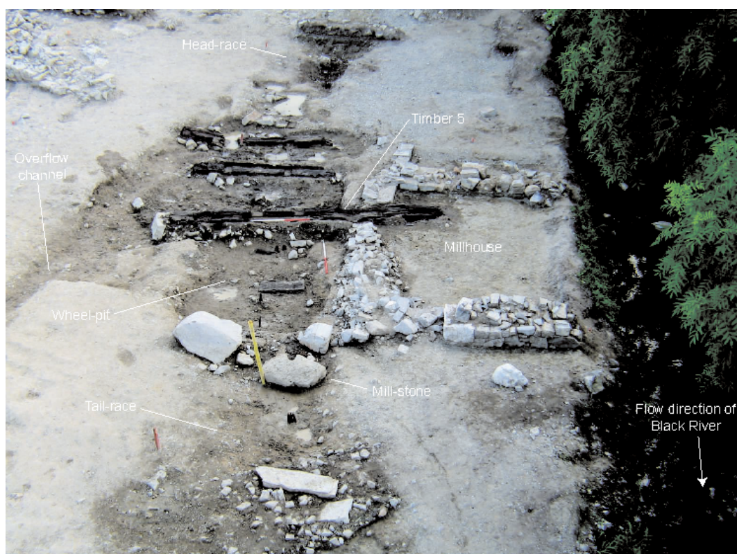
Illus. 9—Elevated view of the vertical watermill (AirShots Ltd).
