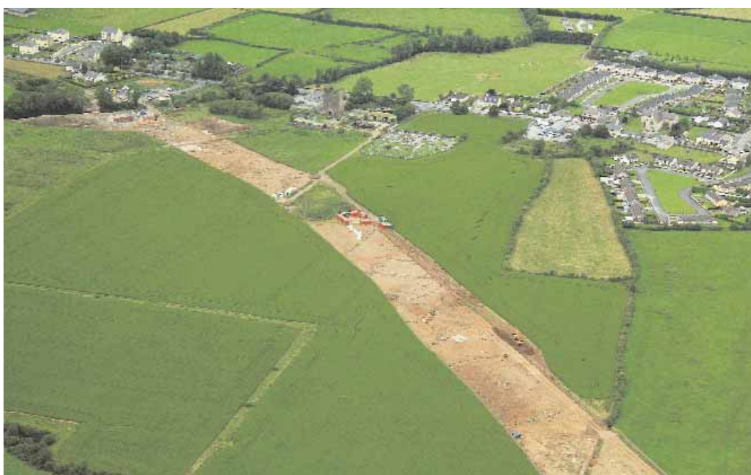
Illus. 2—Aerial view of the excavation area, from the south-east (Studio Lab).
