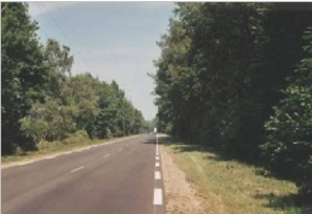
Figure 19 - Limited severity zone, no hard shoulder
