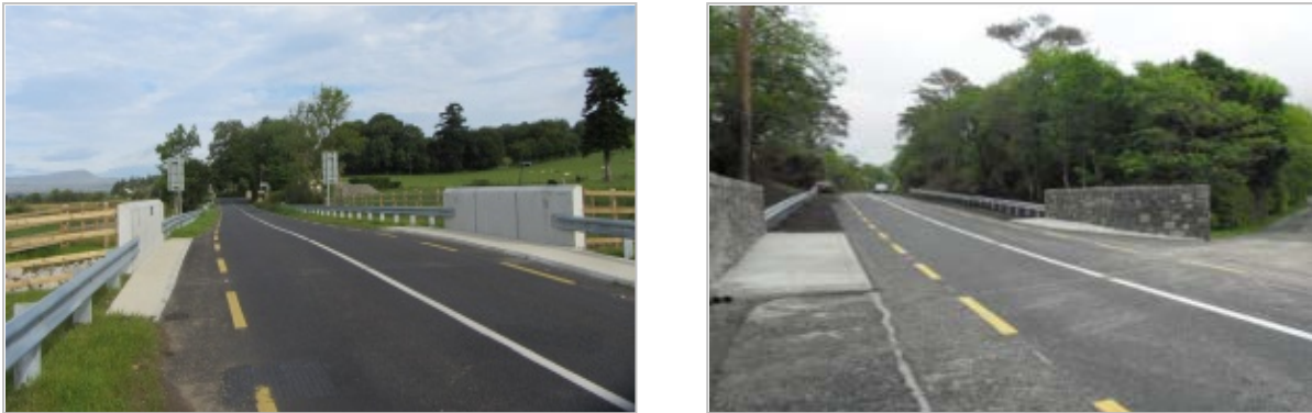
Figure 31 - Transition between semi-rigid and rigid barrier
