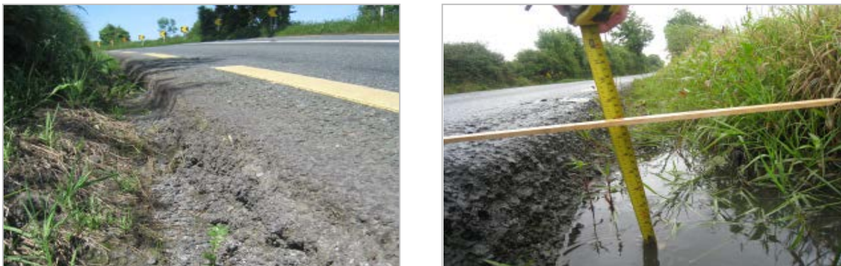
Figure 12 - Pavement-Edge Drop-off
