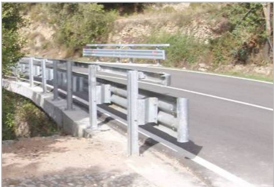
Figure 6 - Examples of hazardous safety barrier terminations
