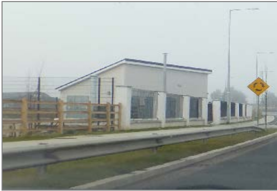
Figure 34 - Typical installations of W-beam semi-rigid barriers
