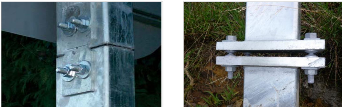
Figure 22 - Breakaway/spliced pole (left) and slip base (right)
