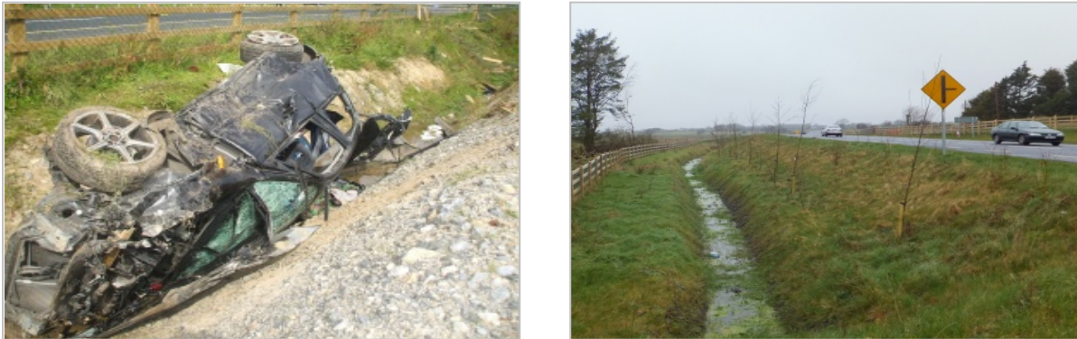
Figure 10 - Examples of hazardous cut (left) and fill slopes (right)
