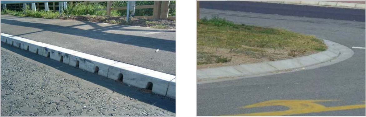
Figure 27 - Vertical kerb (left) and sloping kerb (right)
