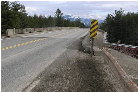
Figure 6 - Examples of hazardous safety barrier terminations
