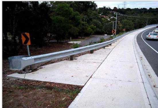
Figure 30 - Deflecting breakaway safety barrier terminal
