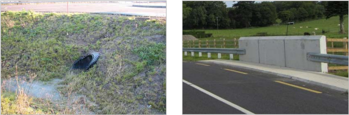
Figure 26 - Bevelled culvert end (left) and parapet (right)
