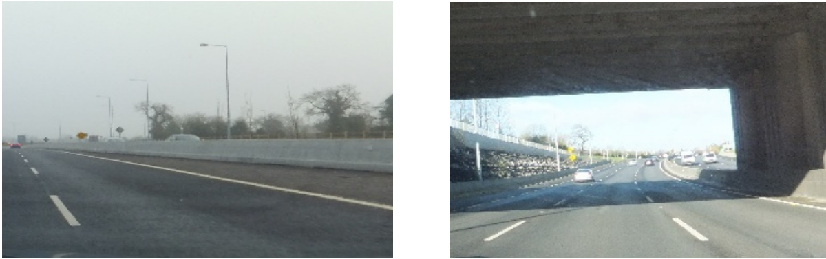
Figure 33 - Examples of rigid median barriers
