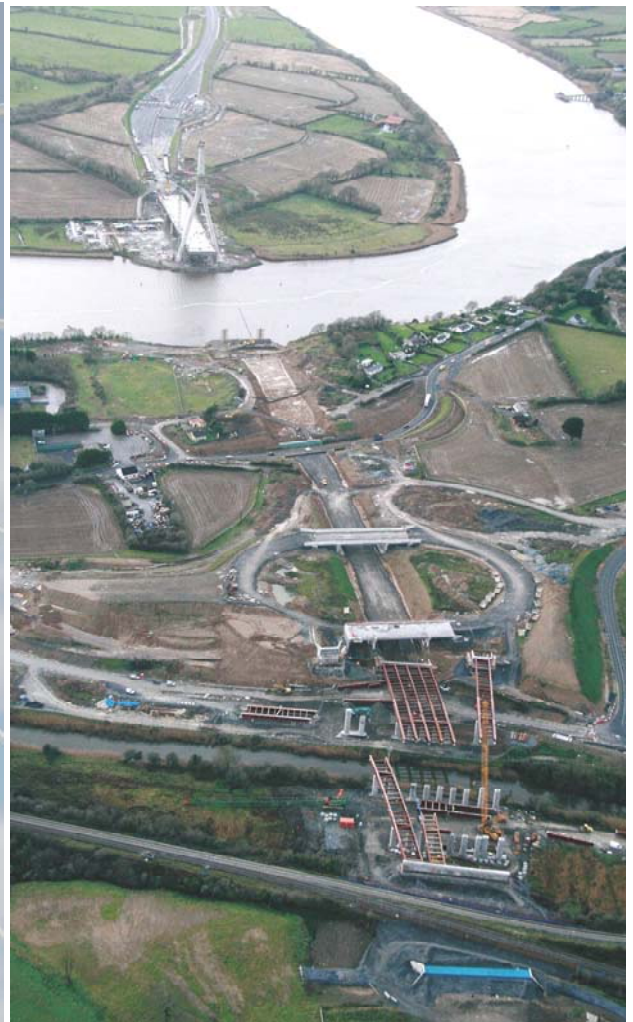
Aerial view of Grannagh Junction & River Suir Bridge under construction
