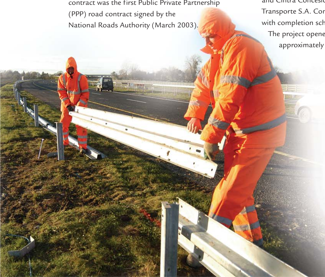
Central Median Safety Barrier A central median safety barrier has been erected and installed over the entire motorway scheme.
