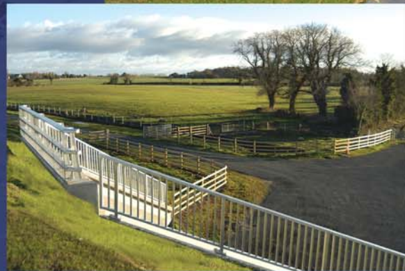
Farm access underpass
