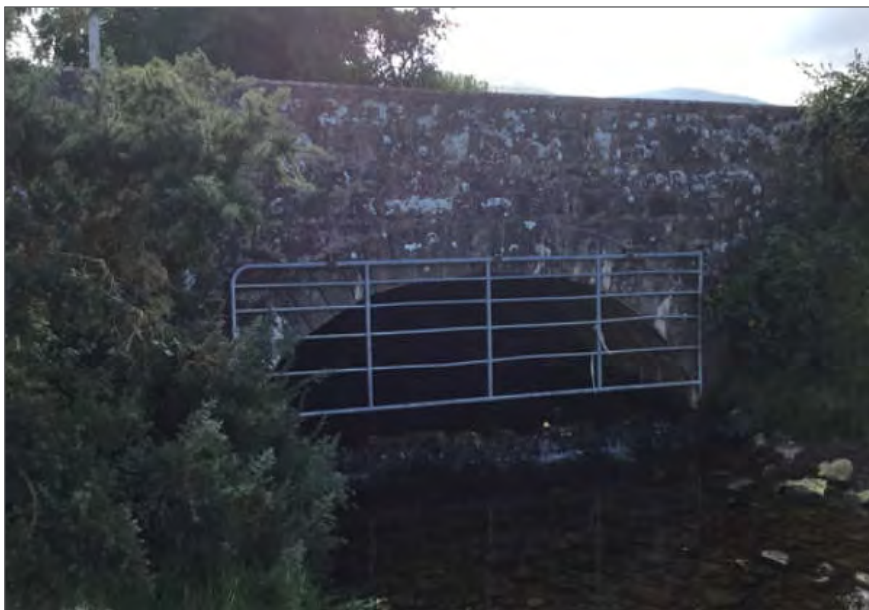
Plate 2-50 Annagh East Bridge.
