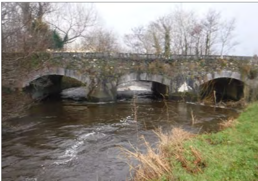
Plate 2-44 River Gweestin Bridge.
