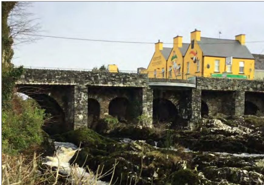
Plate 2-36b Sneem River Bridge.
