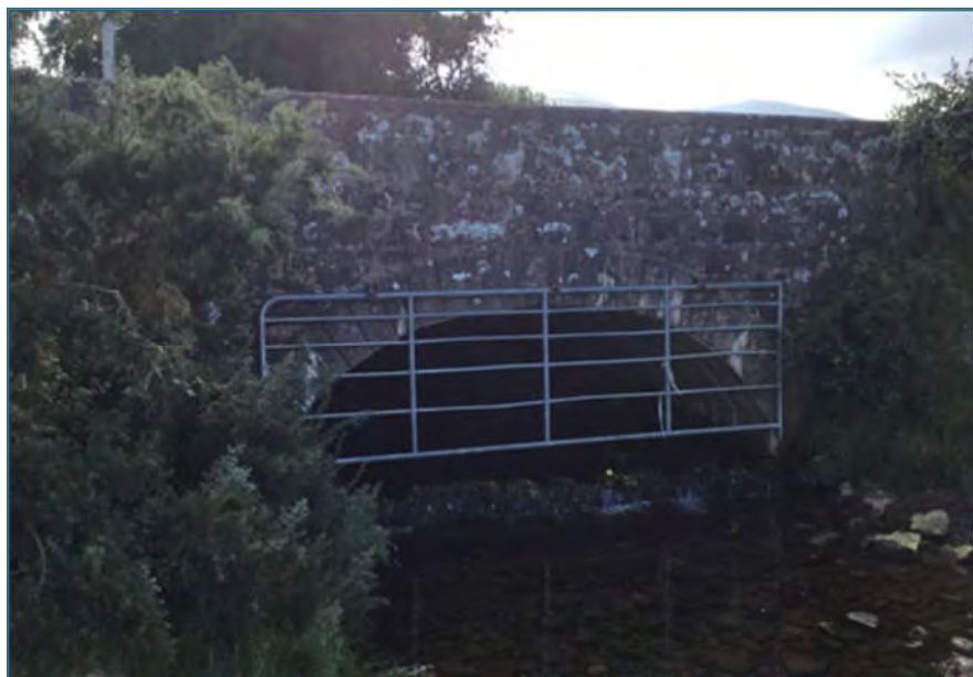
Plate 5-48 Annagh East Bridge.
