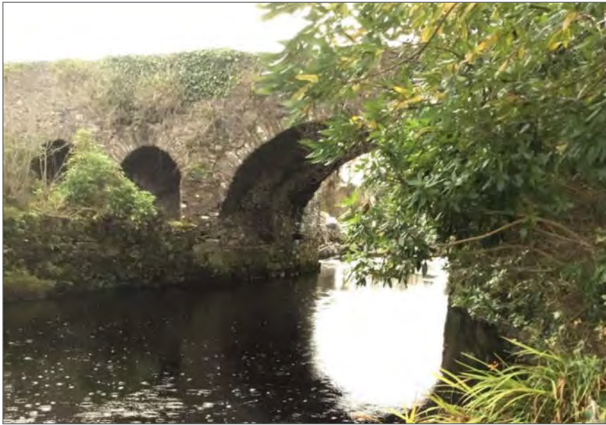
Plate 2-36a Sneem River Bridge.
