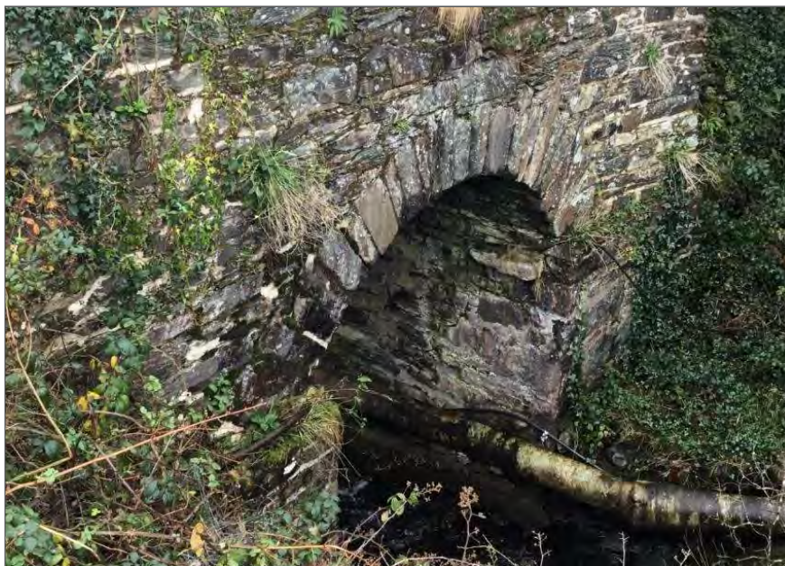
Plate 5-40 Carrig East Bridge.
