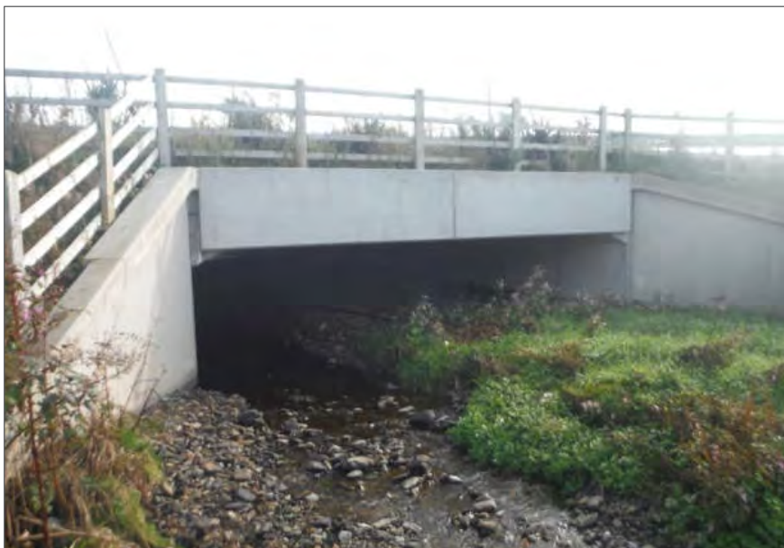
Plate 2-31 Ballybeggan River Bridge.
