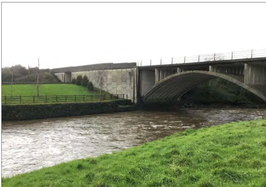
Plate 2-55 Askeaton Friary River Bridge.
