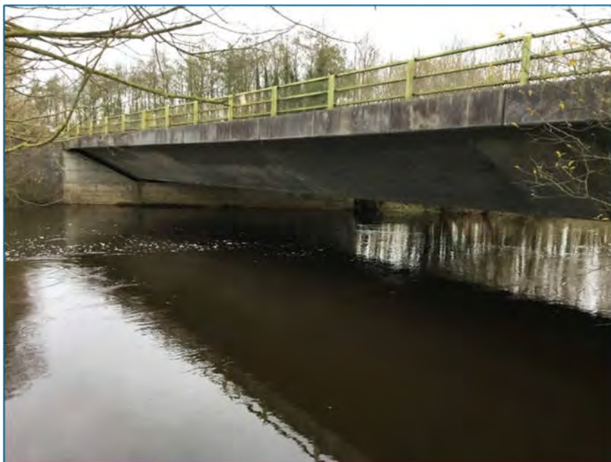
Plate 5-57 Cahirabbey Lower Bridge 1.
