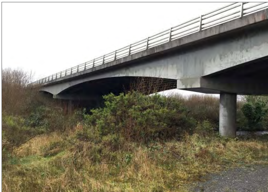
Plate 5-23 River Feale Bridge.
