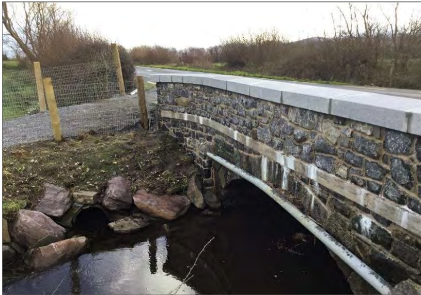
Plate 2-43 Coolroe South Bridge.
