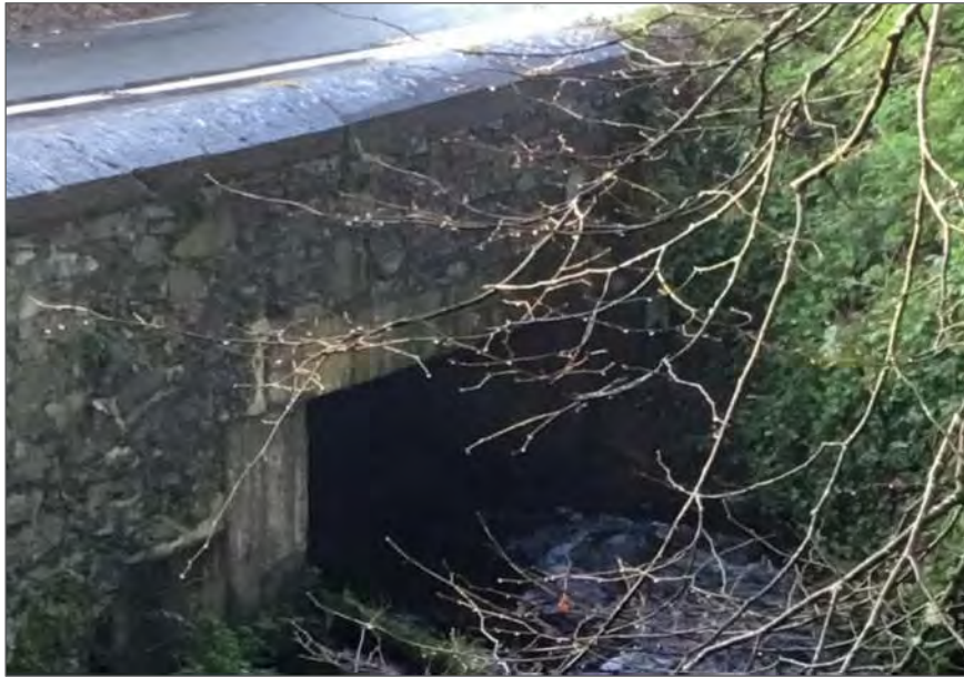
Plate 2-39 Muckcross Friary Bridge.
