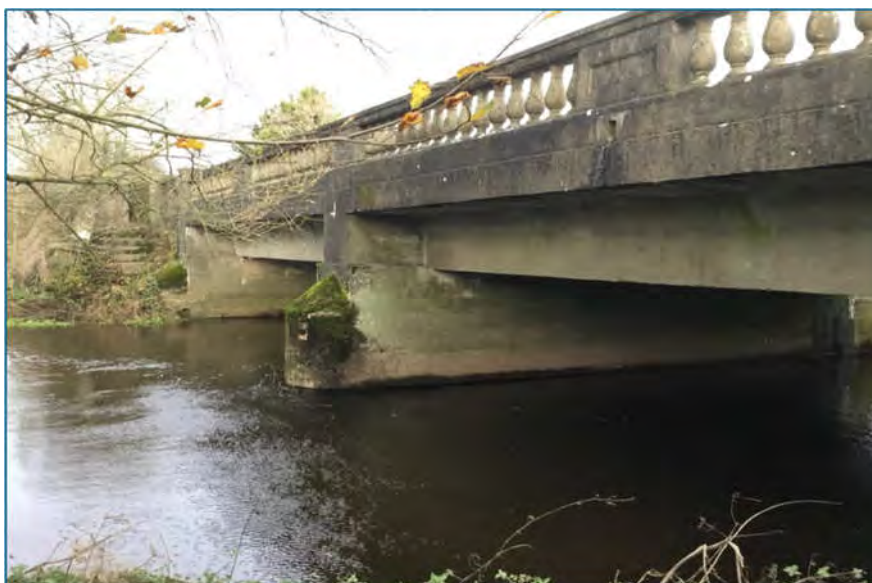
Plate 5-58 Cappa New Bridge.
