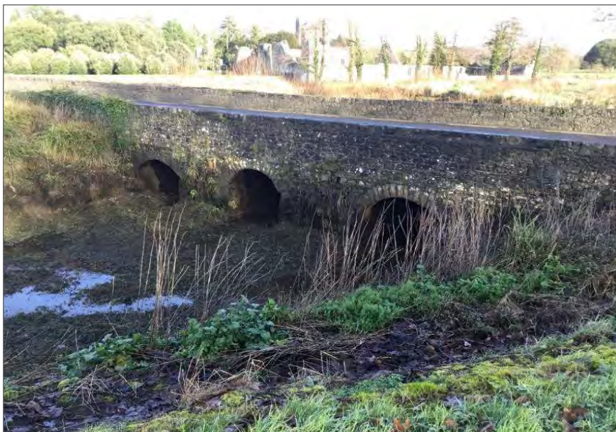
Plate 2-53 Adare Church Bridge.
