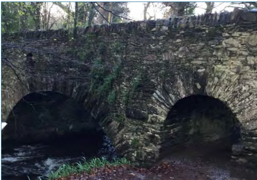
Plate 2-40 Torc New Bridge.
