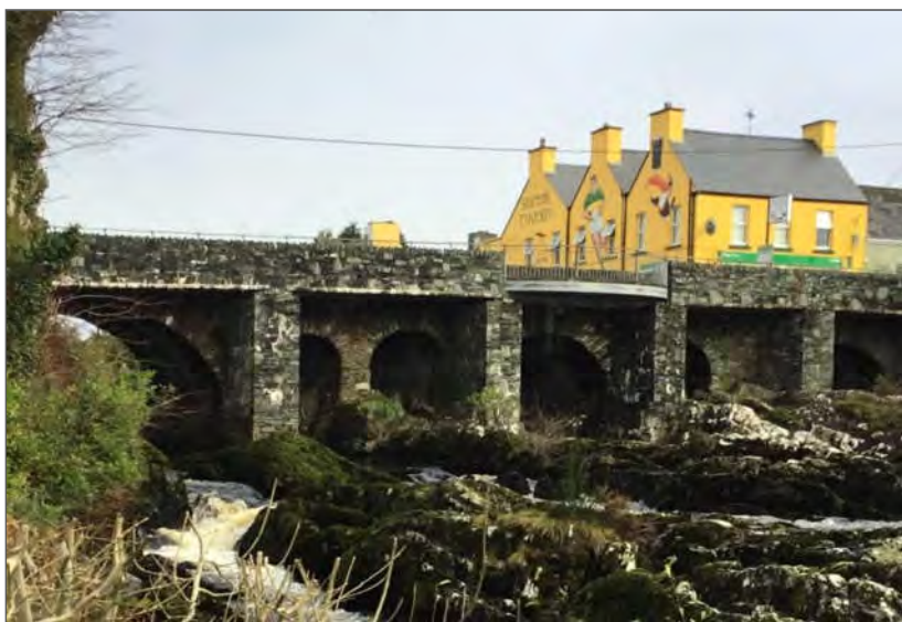
Plate 5-34b Sneem River Bridge.
