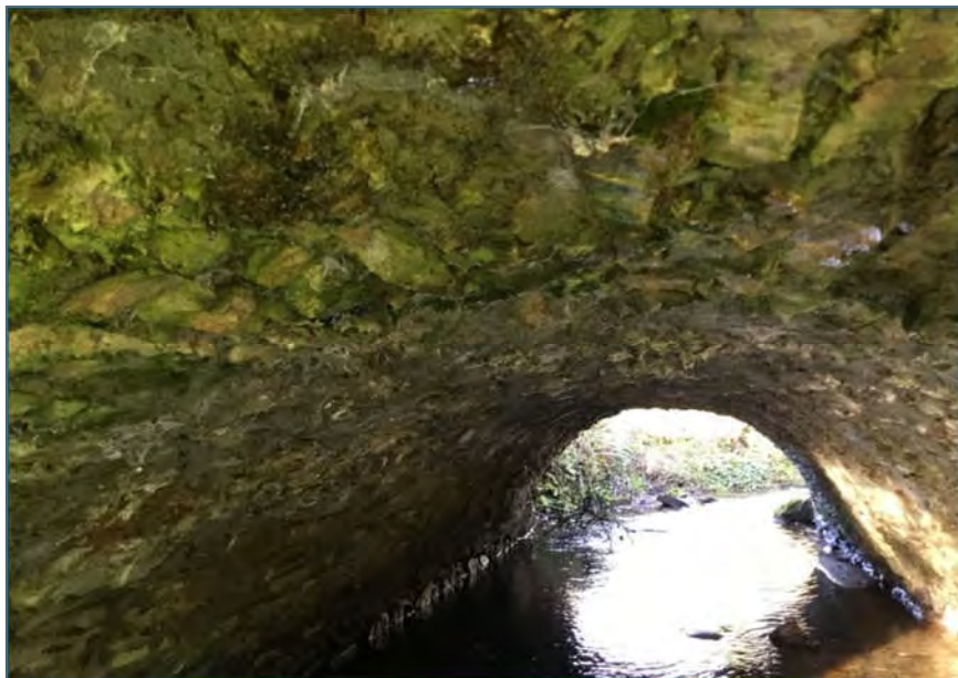
Plate 5-46 Gortanahaneboy West Bridge.
