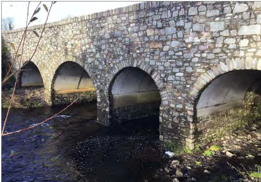
Plate 2-46 Six Mile Bridge.
