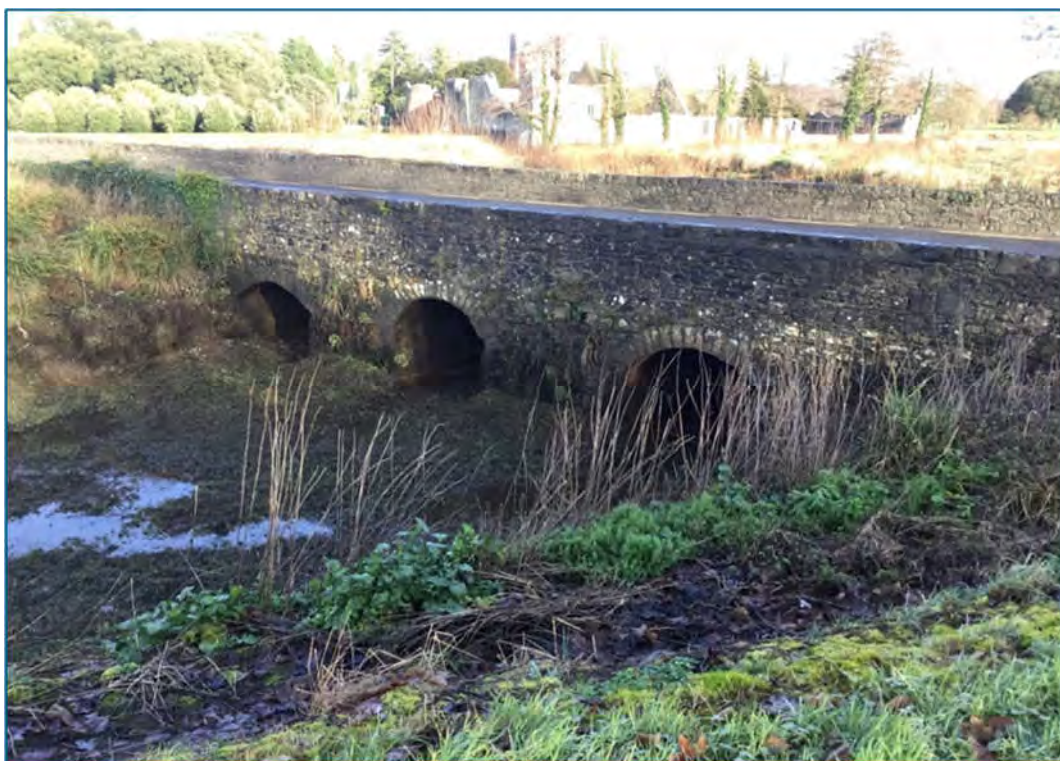
Plate 5-51 Adare Church Bridge.
