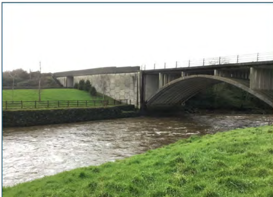
Plate 5-53 Askeaton Friary River Bridge.
