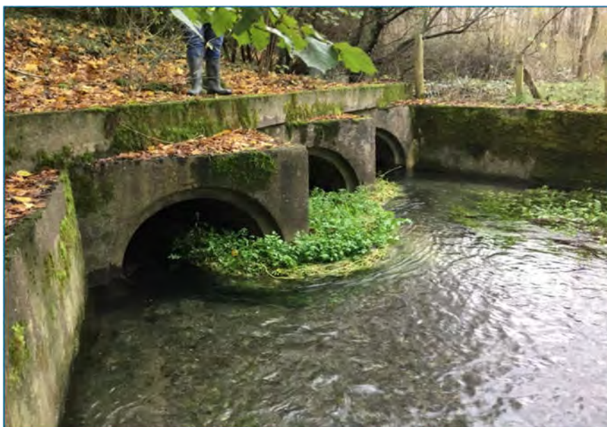
Plate 5-56 Cahirabbey Lower Bridge 2.
