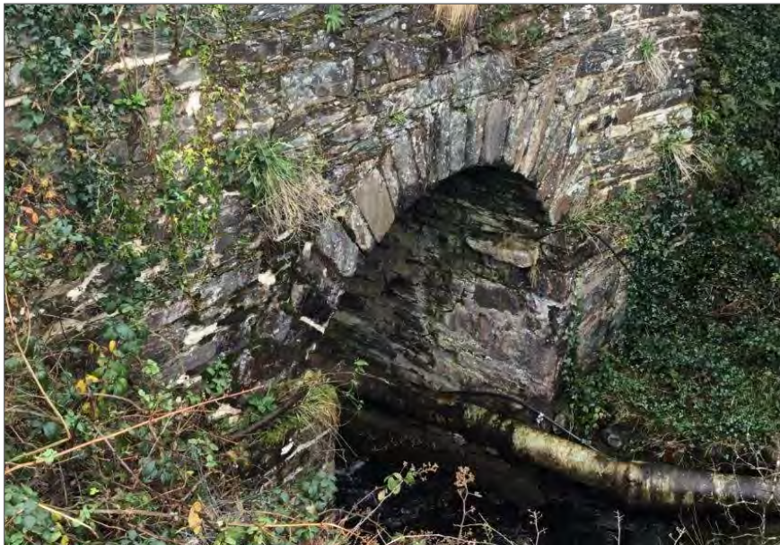
Plate 2-42 Carrig East Bridge.
