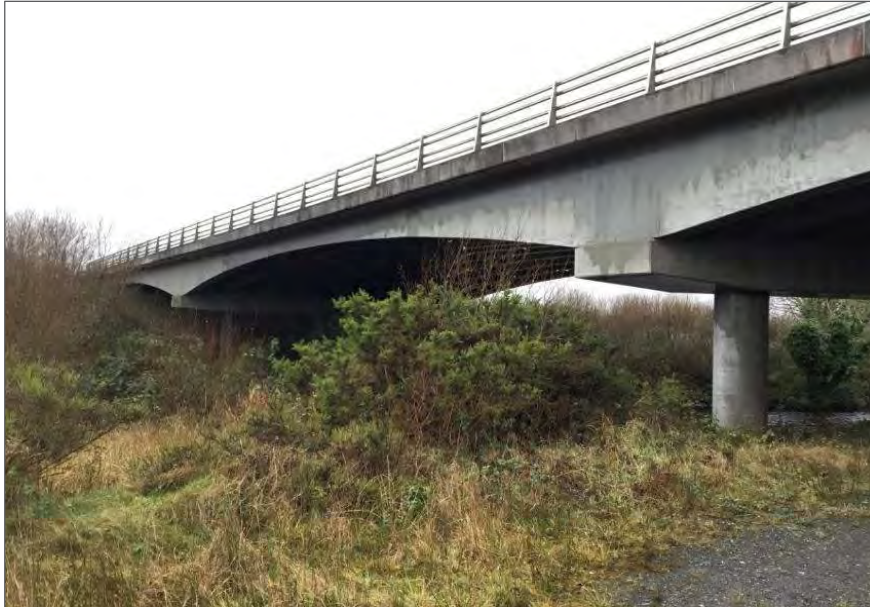
Plate 2-23 River Feale Bridge.
