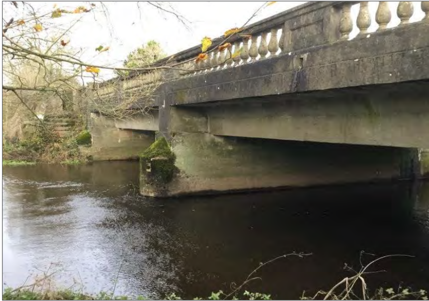
Plate 2-60 Cappa New Bridge.
