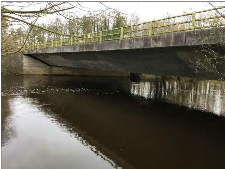
Plate 2-59 Cahirabbey Lower Bridge 2.
