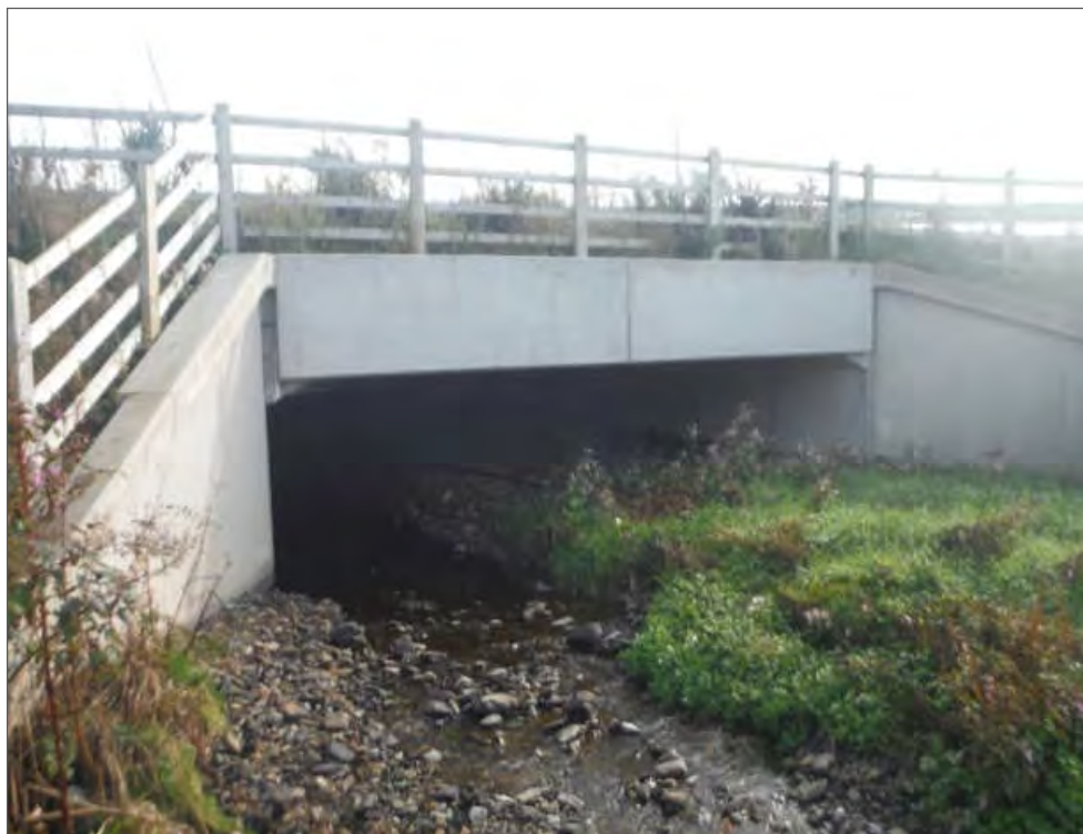
Plate 5-30 Ballybeggan River Bridge.
