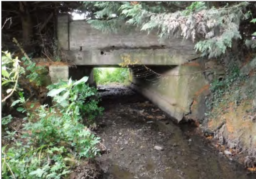
Plate 2-14 Park Road River Bridge, Mallow.
