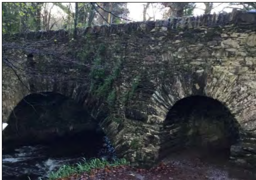
Plate 5-38 Torc New Bridge.
