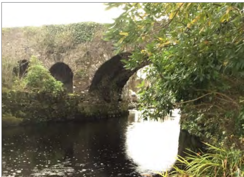
Plate 5-34a Sneem River Bridge.
