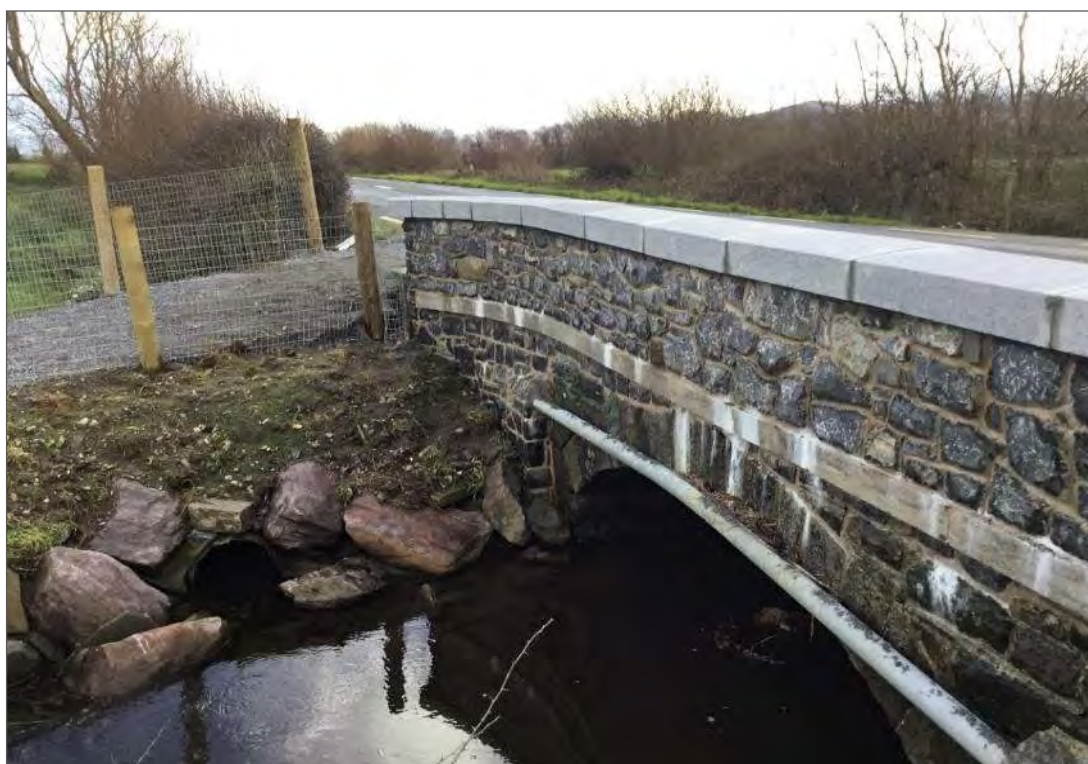
Plate 5-41 Coolroe South Bridge.
