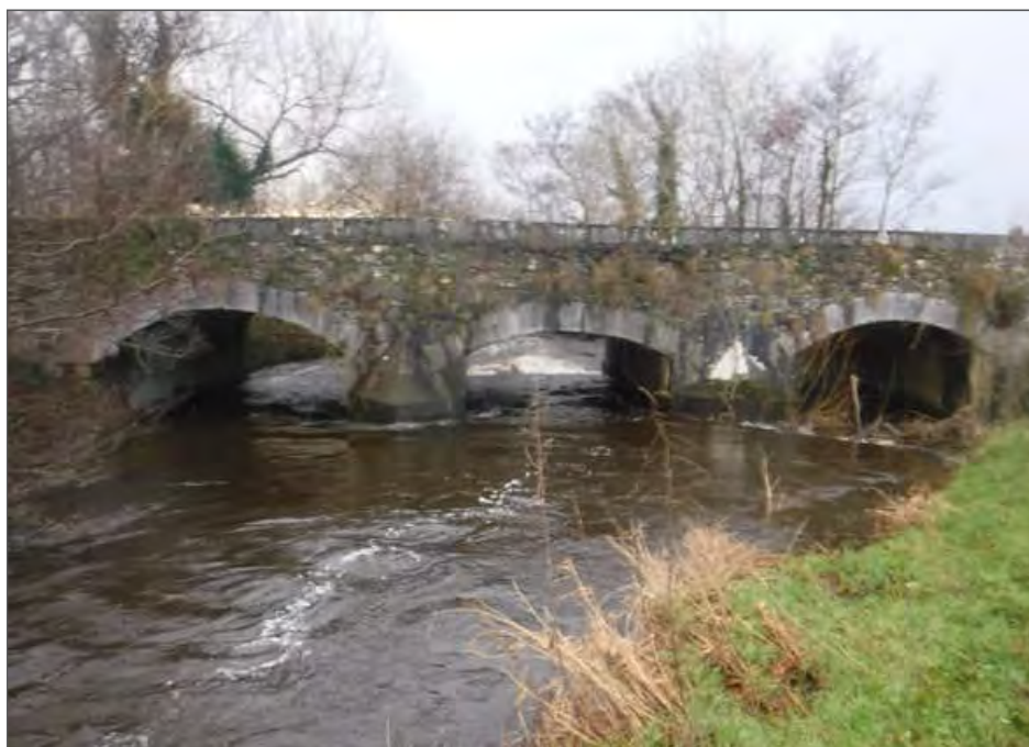
Plate 5-42 River Gweestin Bridge.
