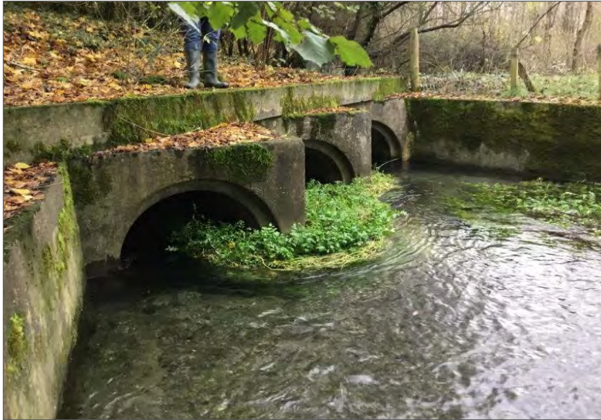
Plate 2-58 Cahirabbey Lower Bridge 2.
