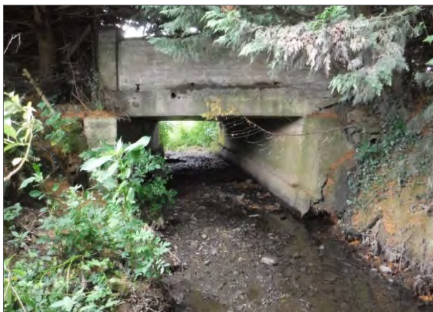
Plate 5-14 Park Road River Bridge.
