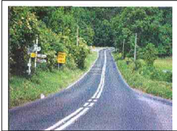
Curly Hole (N51) Western Approach After Accident Remedial Measures were implemented.
