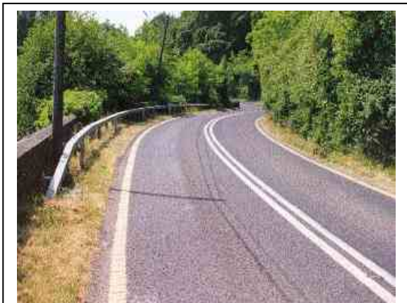
Curly Hole (N51) Eastern Approach. After Accident Remedial Measures were implemented.
