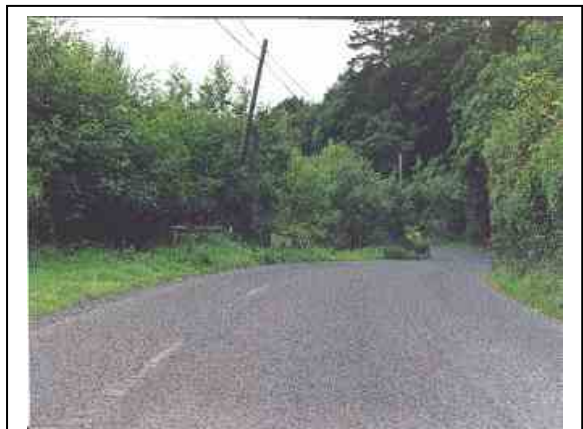
Curly Hole (N51) Eastern Approach. Before Accident Remedial Measures were implemented.
