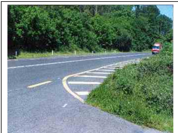
Feede Cross (N1) At Junction looking North. After Accident Remedial Measures were implemented.
