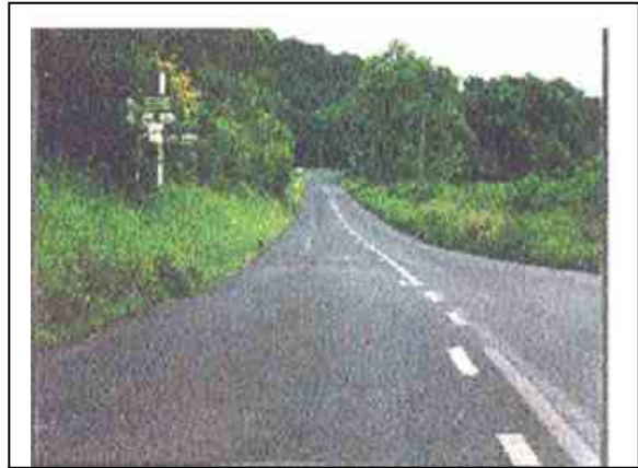
Curly Hole (N51) Western Approach Before Accident Remedial Measures were implemented.
