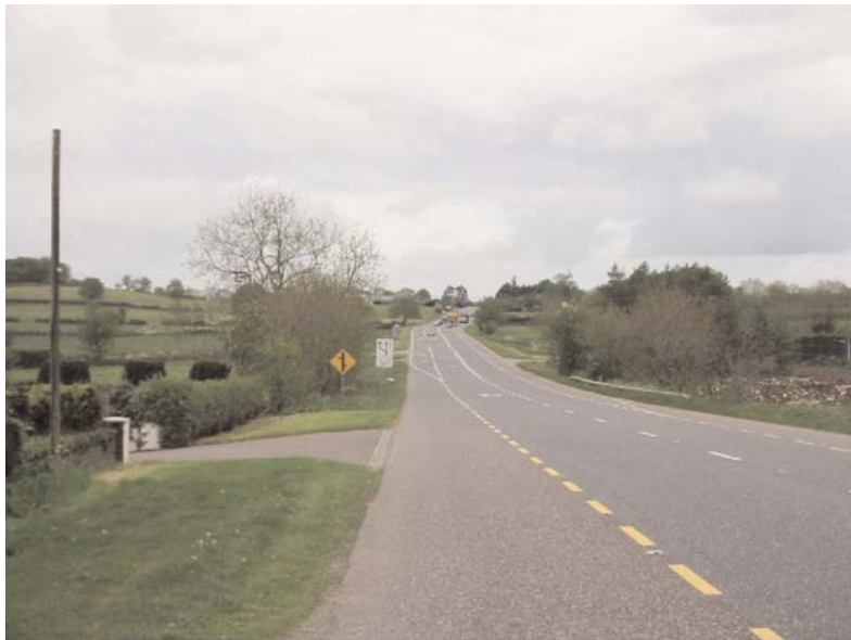
Before road safety remedial measure implemented
