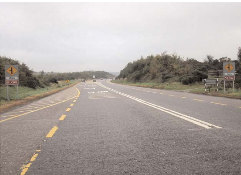
After road safety remedial measure implemented
