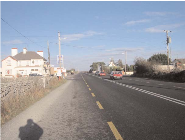
Before road safety remedial measure implemented
