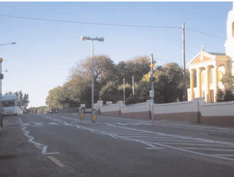
After road safety remedial measure implemented
