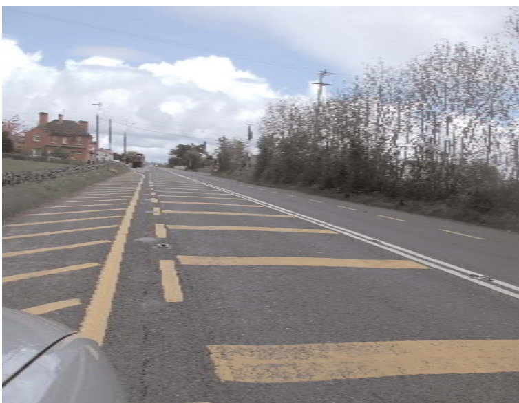
After road safety remedial measure implemented
