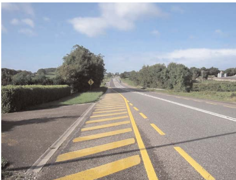
After road safety remedial measure implemented
