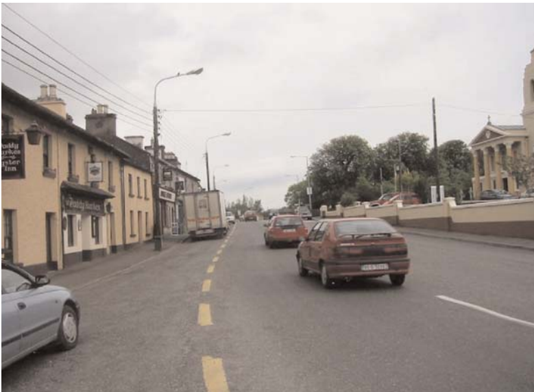
Before road safety remedial measure implemented
