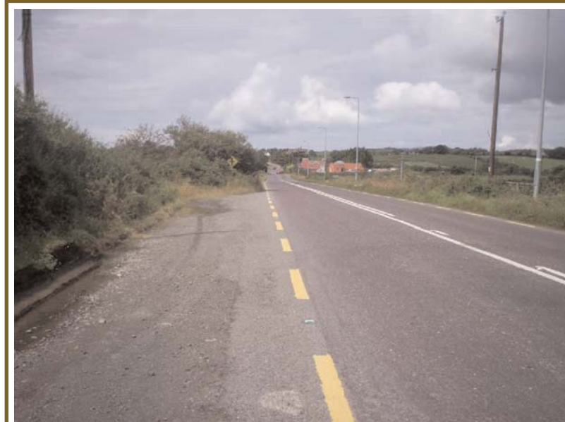
After road safety remedial measure implemented
