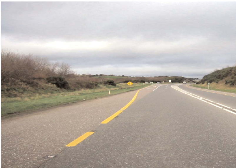
Before road safety remedial measure implemented
