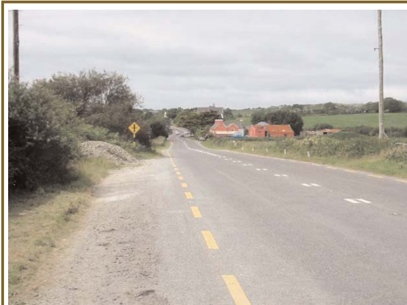
Before road safety remedial measure implemented
