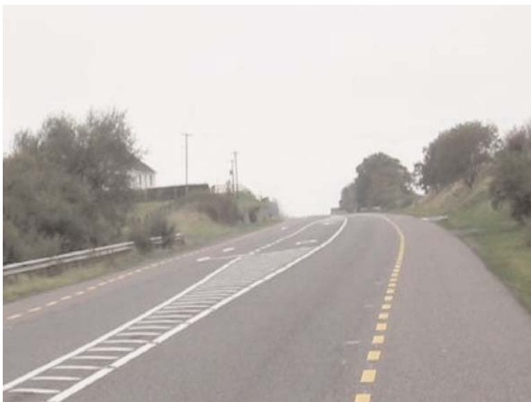
After road safety remedial measure implemented
