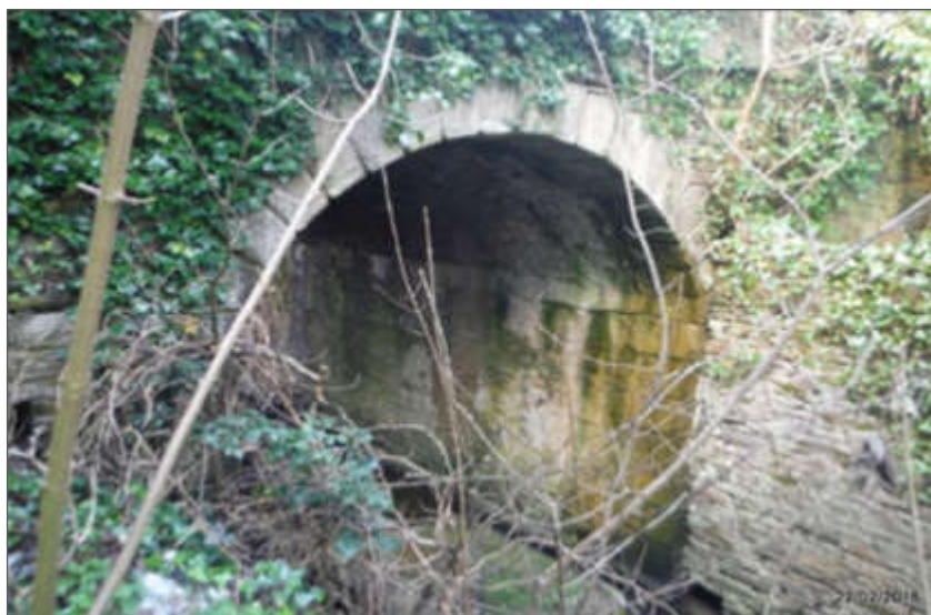
Plate 2-55 Bridge Street Structure Abbeyfeale.
