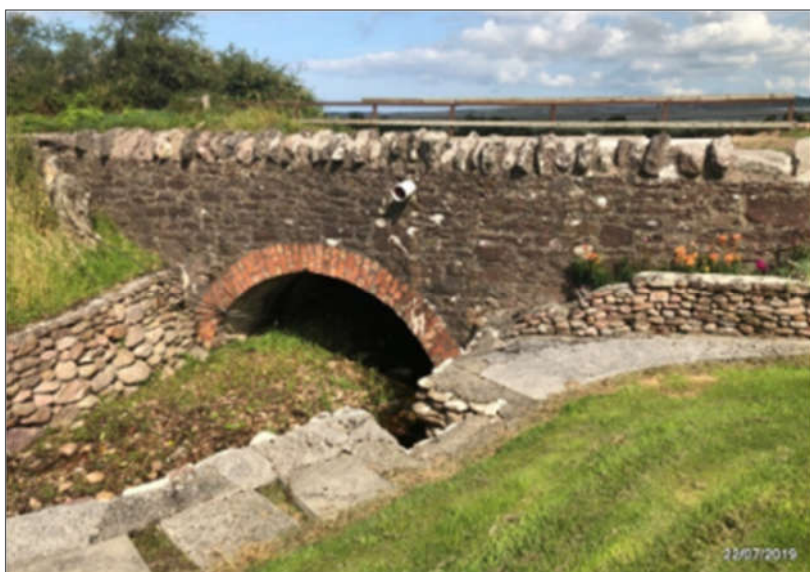
Plate 2-50 The Red Bridge.
