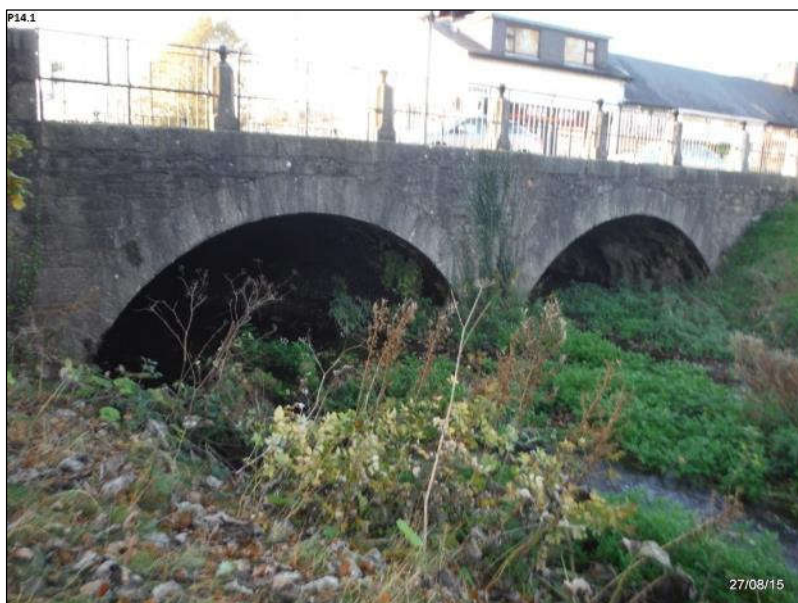
Plate 5-12 Bridge Street Junction, Mallow.
