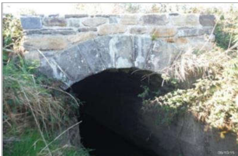
Plate 5-33 Cuss North Culvert.
