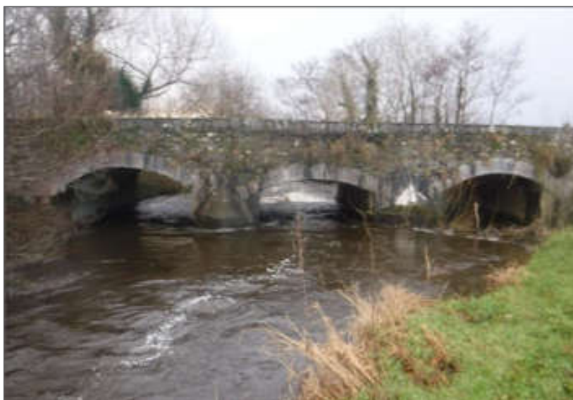
Plate 5-44 River Gweestin Bridge.
