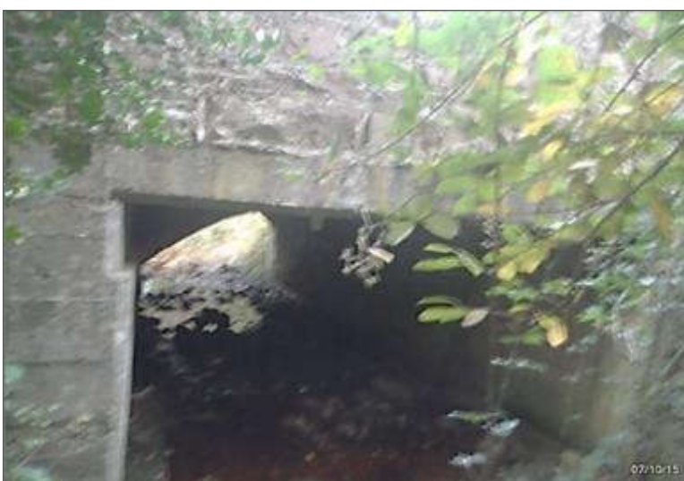
Plate 5-50 Derryquay School West Culvert.
