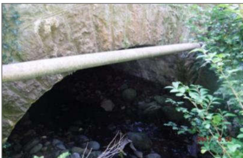
Plate 2-48 Derryquay East Bridge.
