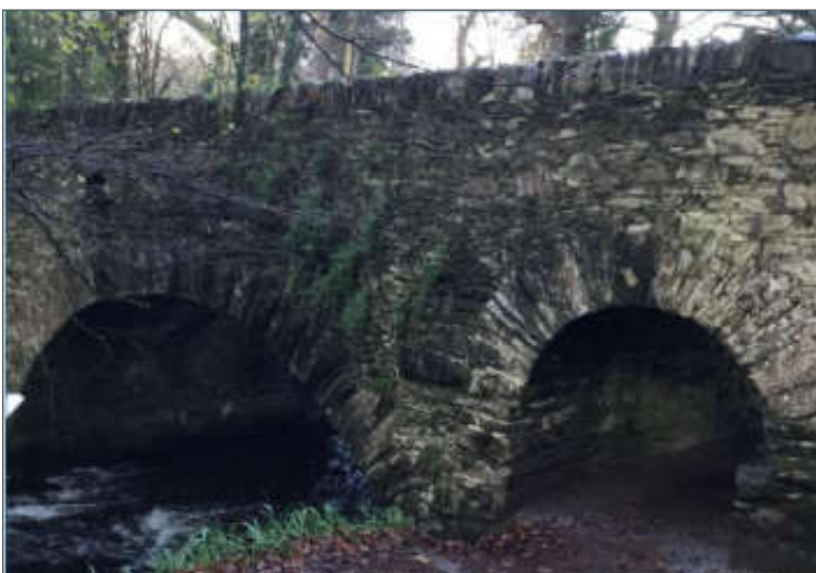
Plate 5-42 Torc New Bridge.
