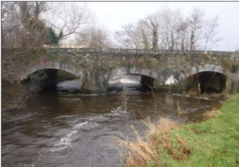
Plate 2-43 River Gweestin Bridge.
