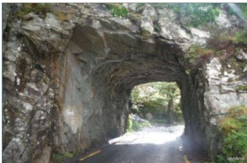
Plate 5-43 Newfoundland Bay Tunnel.
