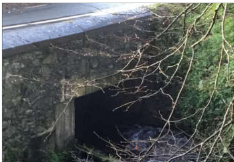
Plate 5-41 Muckcross Friary Bridge.
