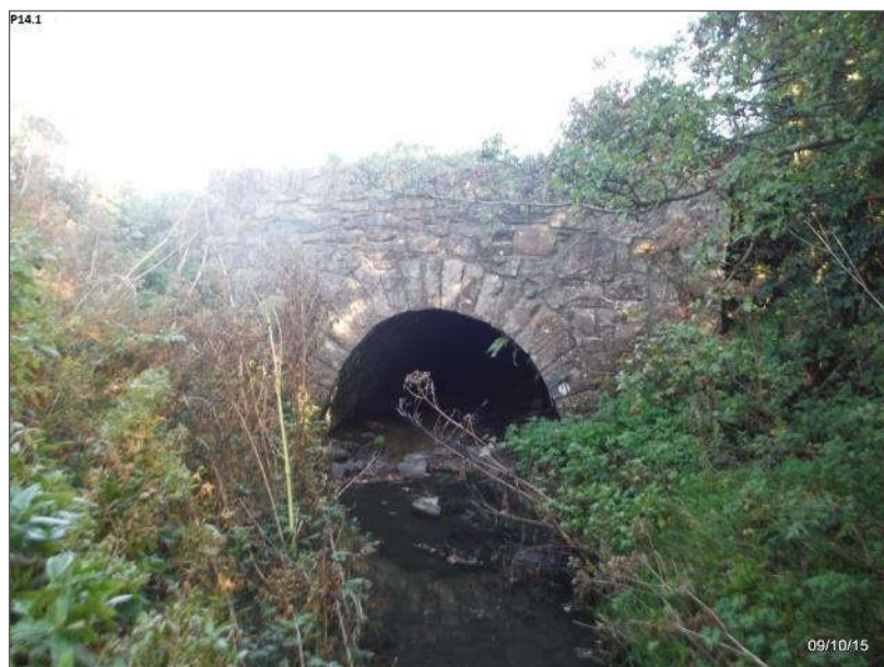
Plate 5-32 Cloontubbrid South Culvert.
