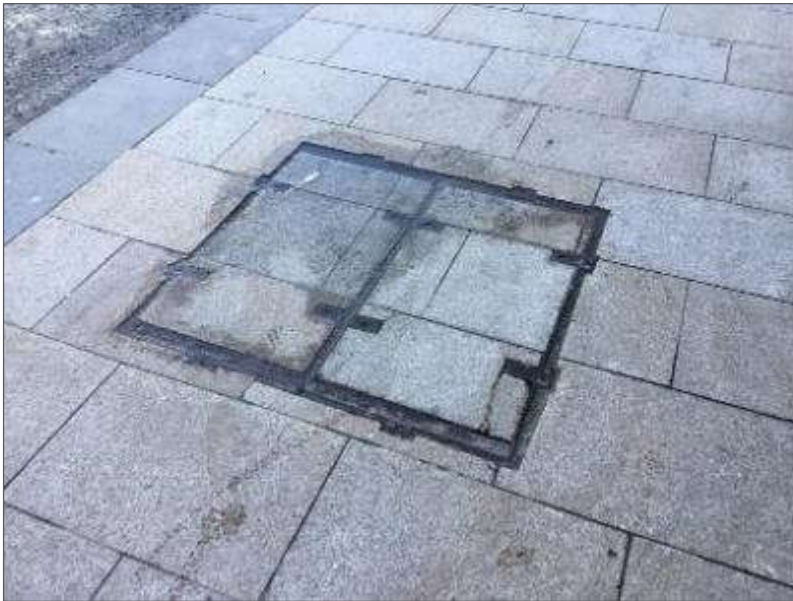
Plate 2-12 Spa Glen Culvert.
