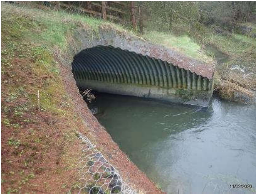
Plate 2-57 Ballysimon N24 Culvert.
