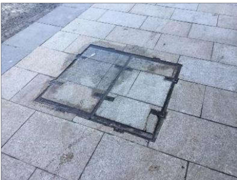
Plate 5-13 Spa Glen Culvert.
