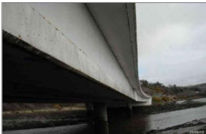
Plate 5-66 Tourig River Bridge.
