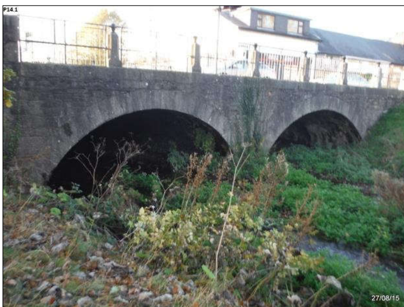
Plate 2-11 Bridge Street Junction, Mallow.
