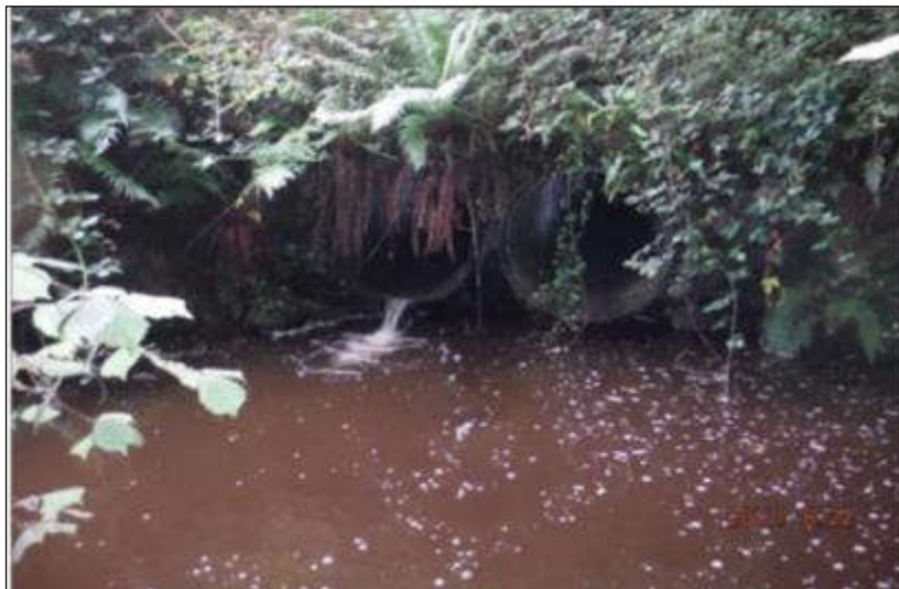
Plate 2-29 Mountcoat Cross Pipe Culvert.
