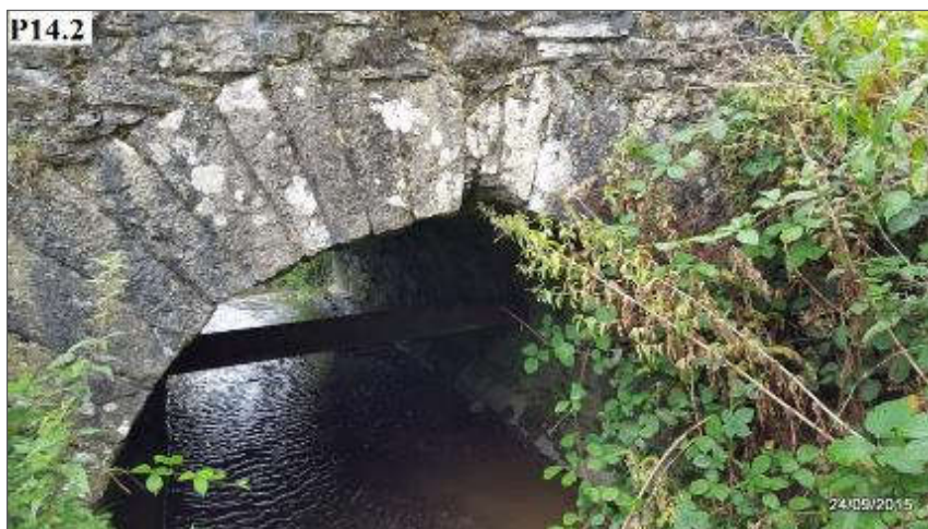
Plate 5-17 Torpys Cross Road Bridge.
