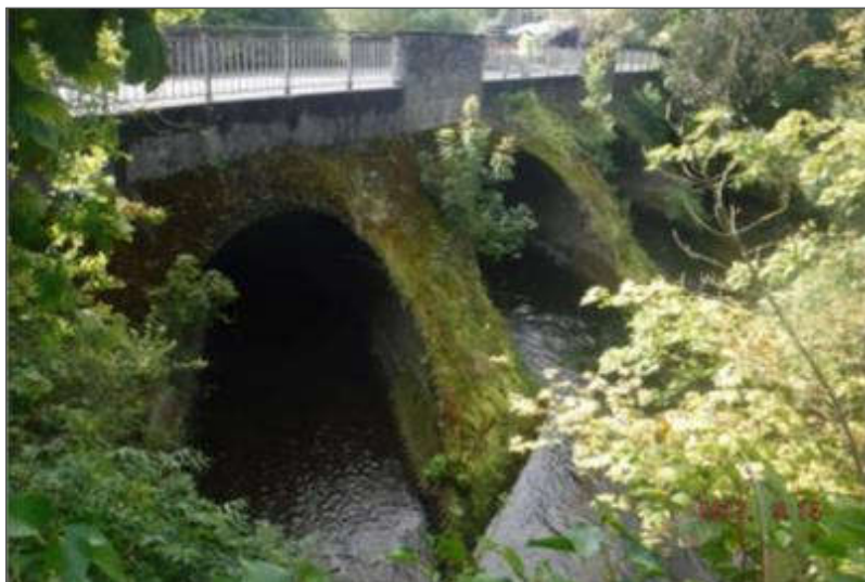
Plate 5-60 Nenagh River Bridge.
