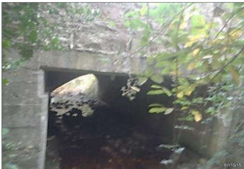
Plate 2-49 Derryquay School West Culvert.
