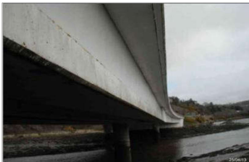
Plate 2-65 Tourig River Bridge.
