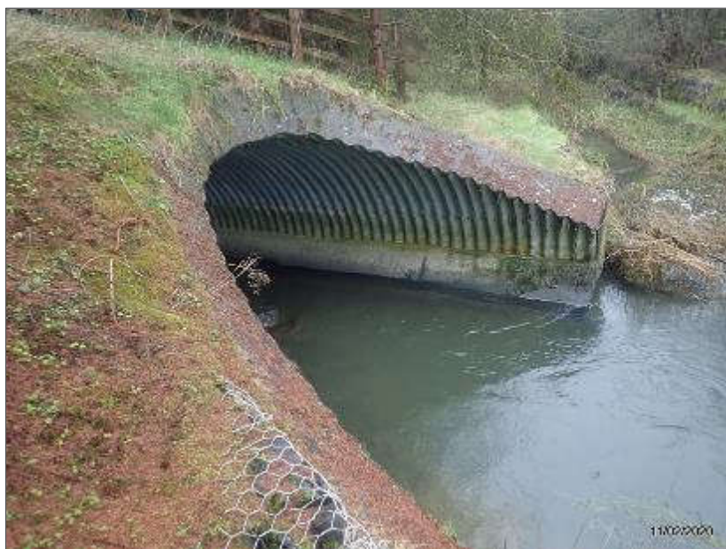
Plate 5-58 Ballysimon N24 Culvert.
