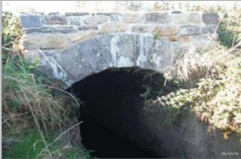
Plate 2-32 Cuss North Culvert.
