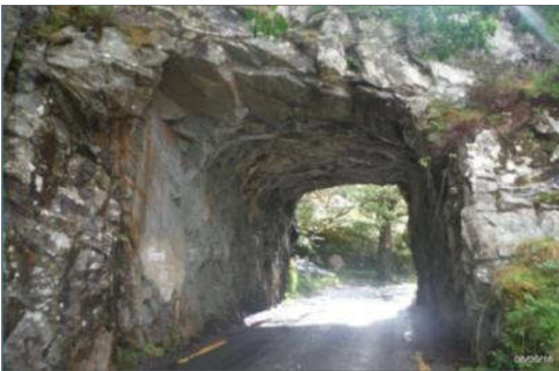
Plate 2-42 Newfoundland Bay Tunnel.
