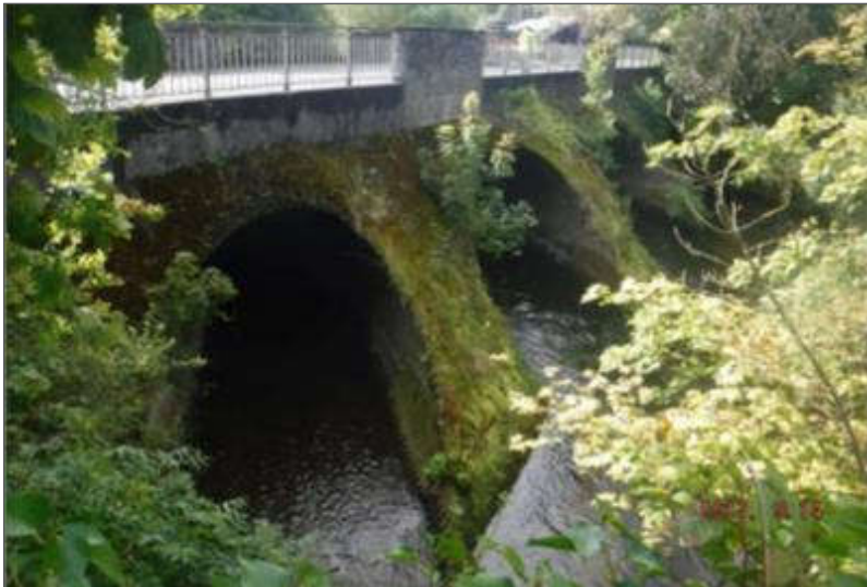
Plate 2-59 Nenagh River Bridge.
