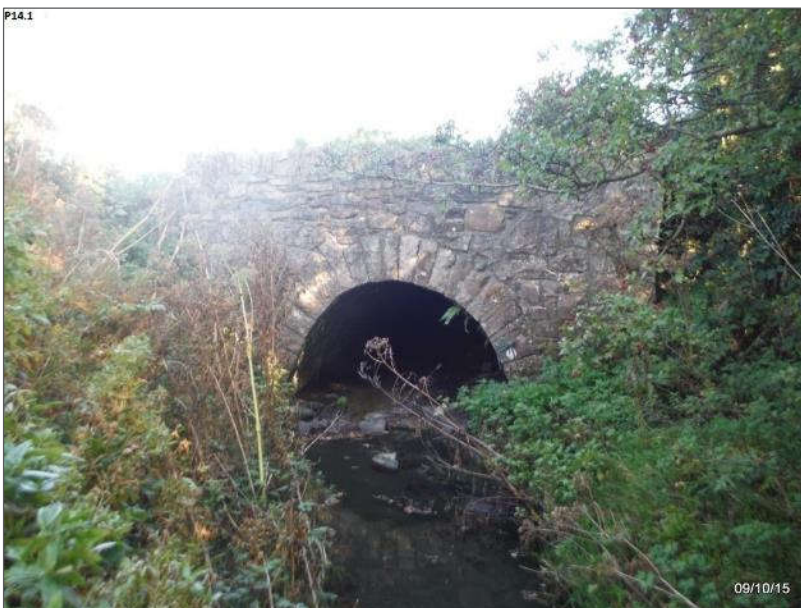
Plate 2-31 Cloontubbrid South Culvert.
