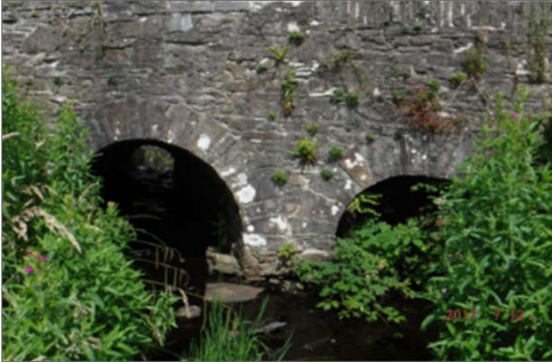
Plate 2-21 Liscasey Bridge West.
