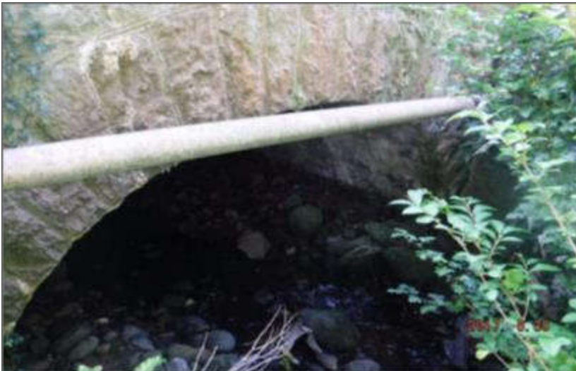
Plate 5-49 Derryquay East Bridge.
