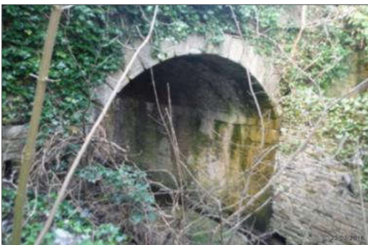
Plate 5-56 Bridge Street Structure Abbeyfeale.
