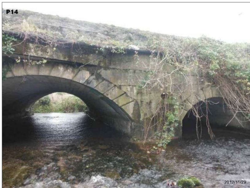
Plate 2-64 Old Pike Bridge.
