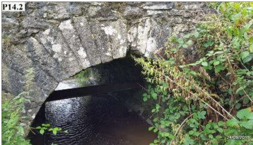
Plate 2-16 Torpys Cross Road Bridge.
