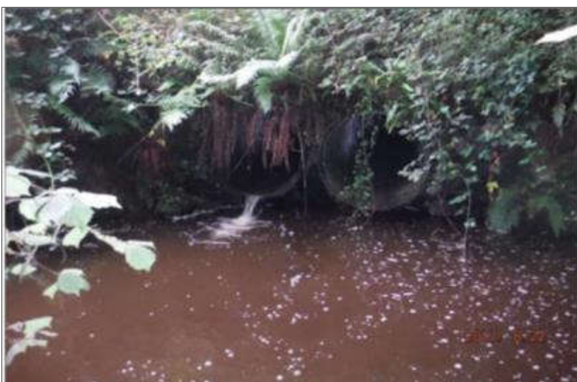
Plate 2-30 Mountcoat Cross Pipe Culvert.
