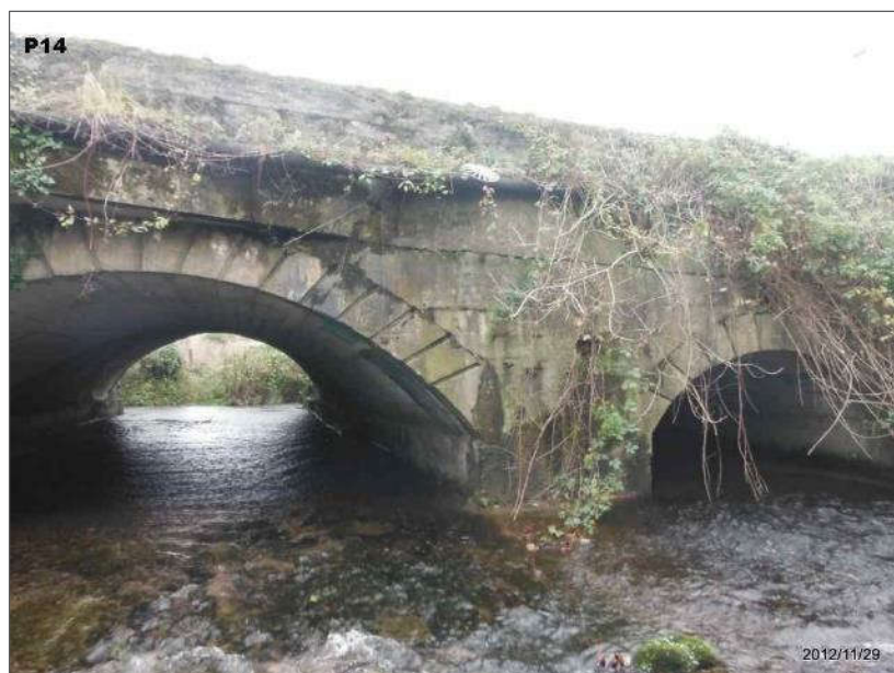
Plate 5-65 Old Pike Bridge.
