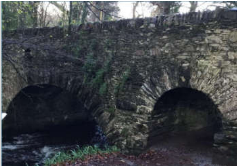
Plate 2-41 Torc New Bridge.
