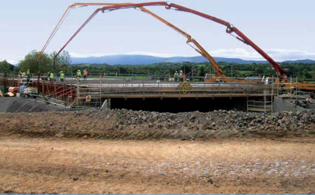
➤ Pouring of Bridge Deck
