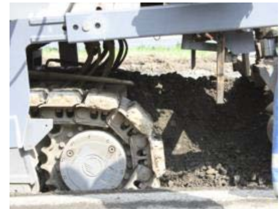
Cold in-situ recycling by DCR machine
