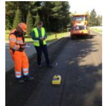
Compaction check by Troxler sensor head
