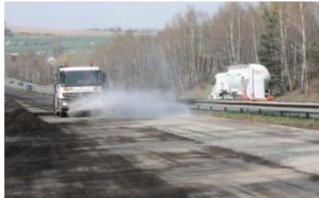
Water spraying on fresh CR
