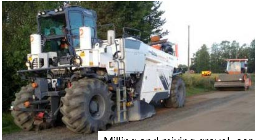
Milling and mixing gravel, asphalt top layer and unbound material
