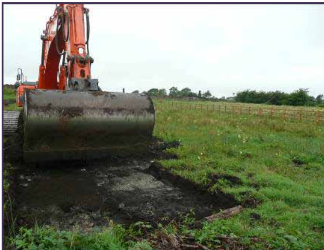
Figure 5: Stripping of wet grassland (GS4) soils (Photograph courtesy of Lisa M.J Dolan)
