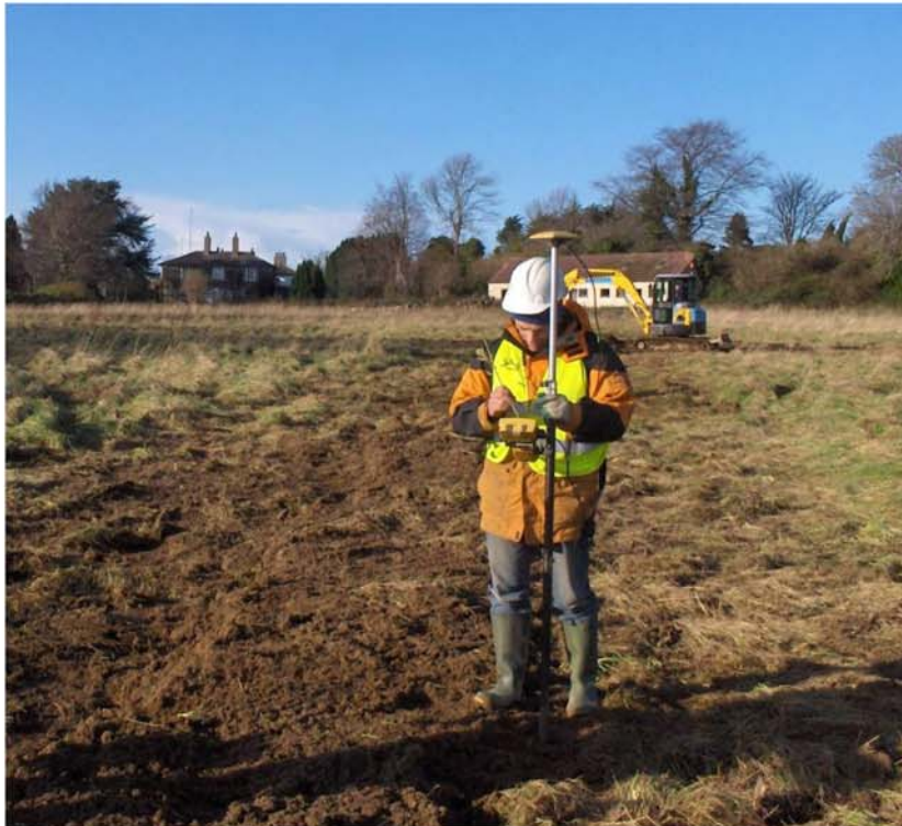
Plate 9: Ian Elliott surveying in test trenches with GPS
