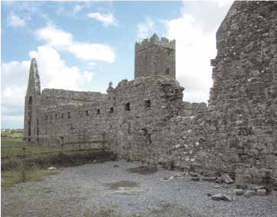
Illus. 3—The roughly surfaced carpark prior to the excavations (TVAS [Ireland] Ltd).
