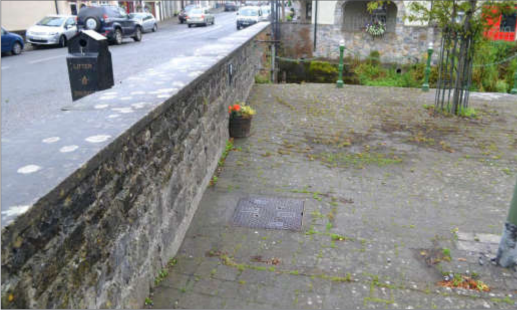
Plate 4.5 Existing manhole access to the culvert (from RPS, 2017).
