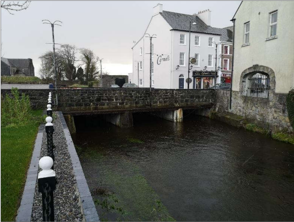
Plate 4.3 West elevation of main bridge, Ballyfinboy River (February, 2022).
