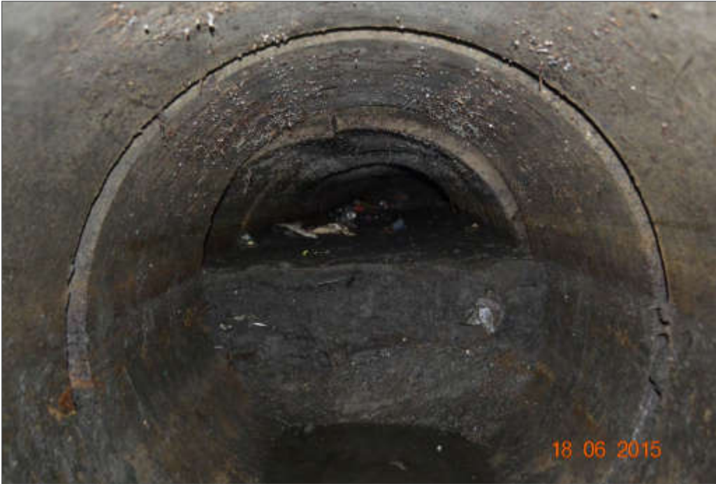
Plate 4.9 View through the culvert (from RPS, 2017).
