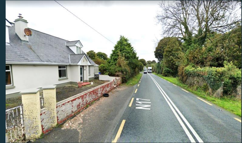
Existing N17 Legacy Network (Sub-standard Cross Section and hazards at edge of carriageway)
