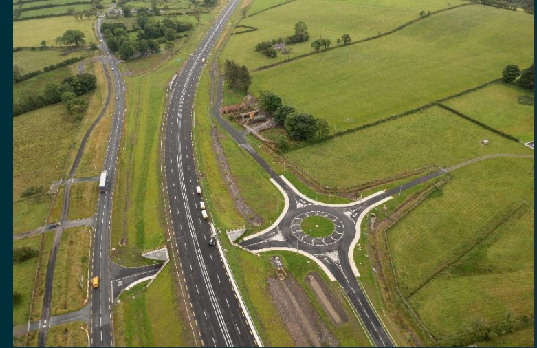
N4 Realignment at Doorly Td.
