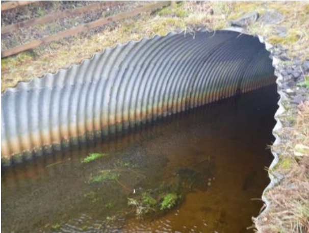
Figure 3-1 - Boherduff culvert entrance
