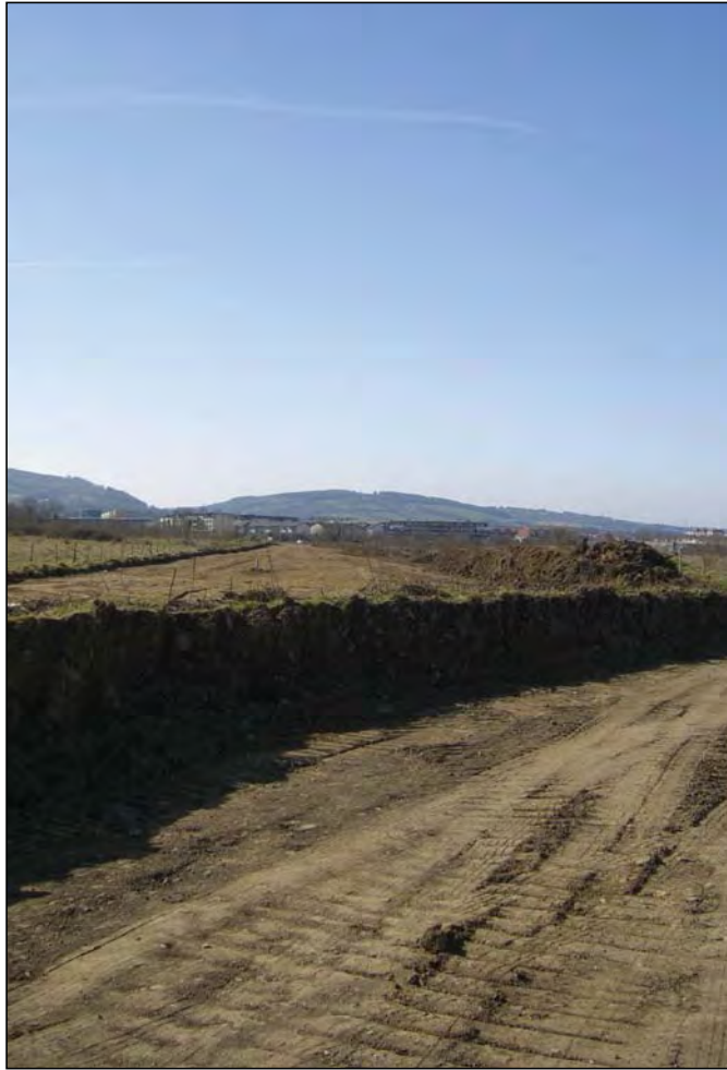
Plate 3. Testing area 2. CityWest Campus
