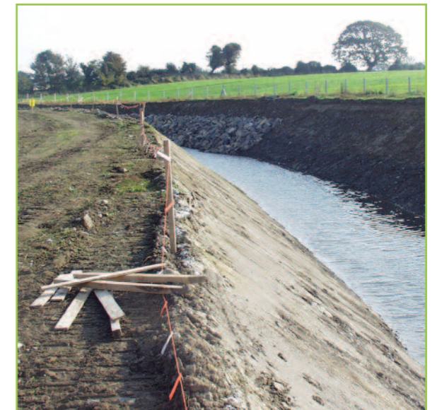
A poor example of a realigned watercourse with a highly uniform trapezoidal profile and flow regime. This limits the ecological potential of the river as well as reducing landscape quality through a "loss of naturalness" within the landscape.
