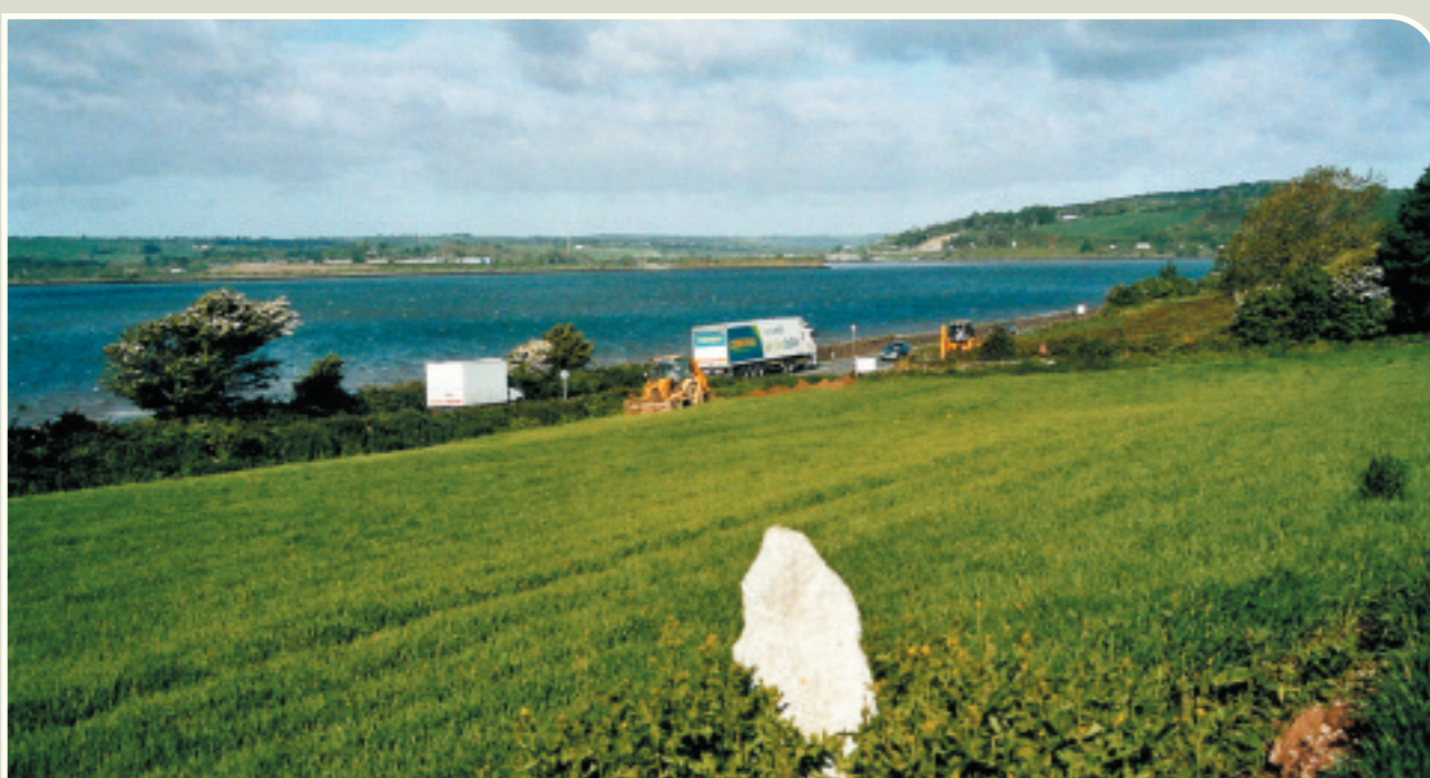
View of road works from standing stone at Shanacoole. (RMP WA037-052)
