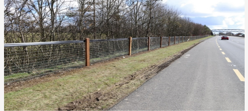
Repairs to Mesh fence following collision 2
