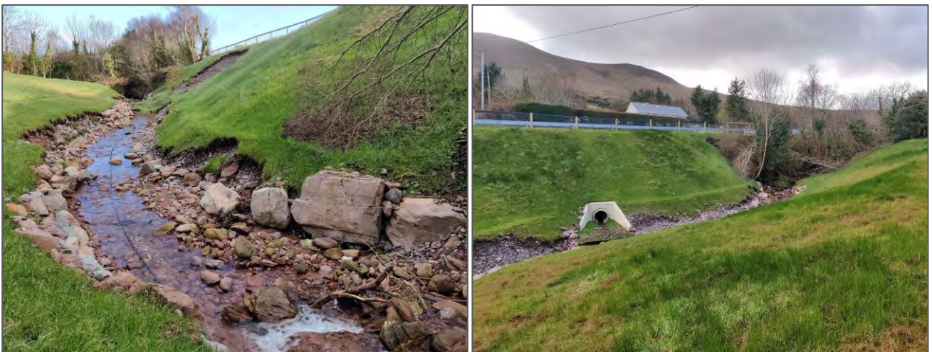
Figure 4-3 - Overview of the main works area (January 2024).
