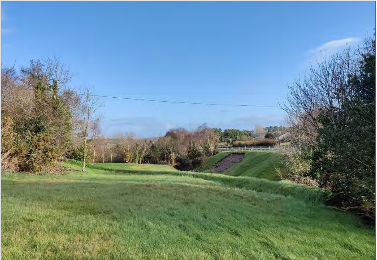
Figure 4-2 - View east along access to the main works area (January 2024). Note earth bank intercepting any run-off from the compound area to the stream.
