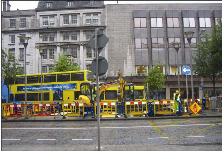
Plate 1 - Pre-excitation of ST709, O'Connell St., west-facing.
