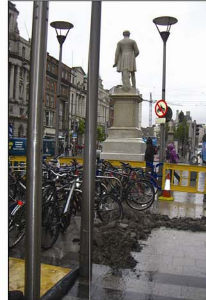
Plate 4 - Mid-excitation of ST711 and ST712, north-facing.
