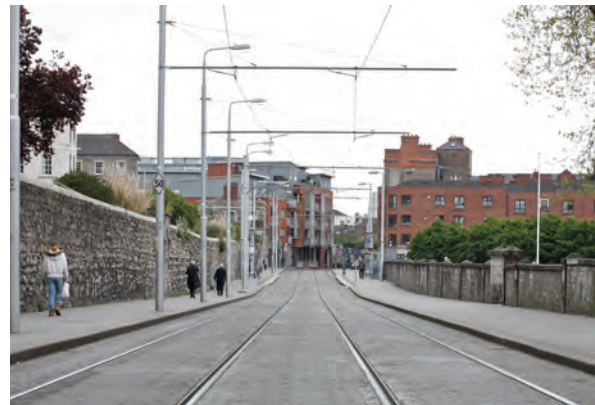
Photo 1.4 Embedded track on the Luas Red Line
