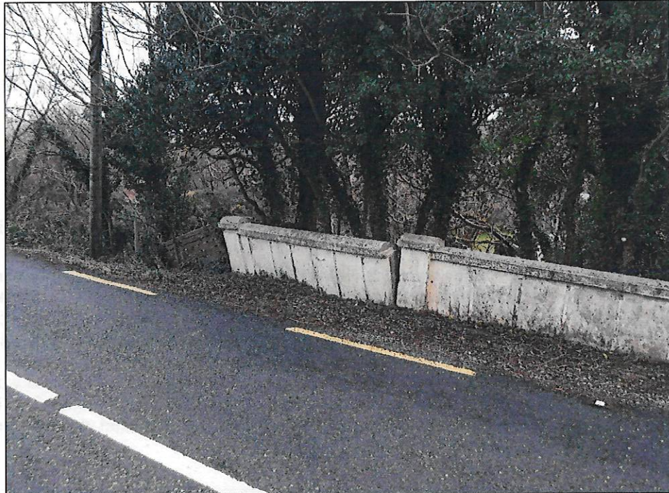
Plate 1. Letterfore bridge, parapet wall (a) [Source: Atkins R.E.; 16/01/2019]
