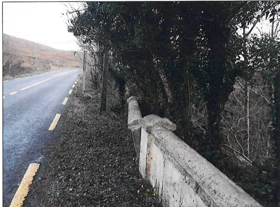
Plate 2. Letterfore bridge, parapet wall (b) [Source: Atkins R.E.; 16/01/2019]
