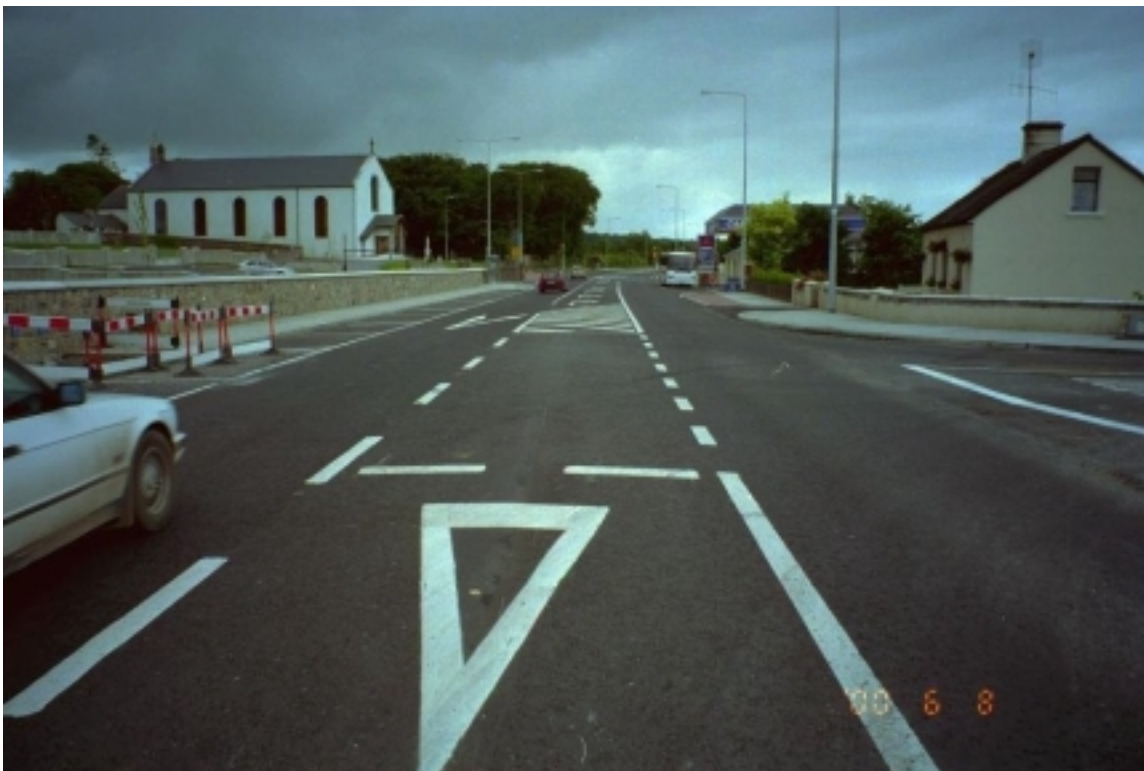
Photo 7: N20 Ballyhea, Co. Cork – Staggered Junction ‘after’
