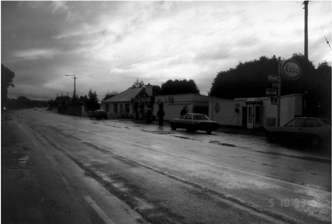
Photo 6: N20 Ballyhea, Co. Cork – Staggered Junction ‘before’
