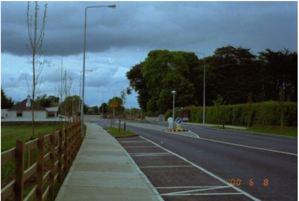
Photo 8: N20 Ballyhea, Co. Cork – Buildouts, Parking and Bus Bay ‘after’
