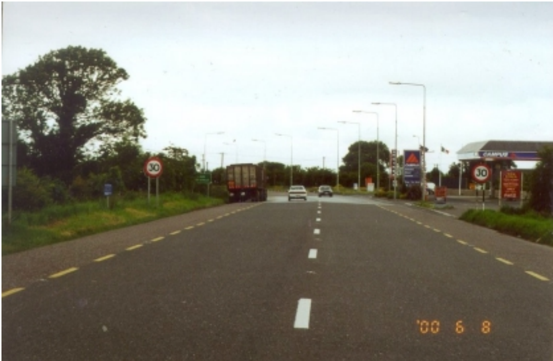
Photo 1: N20 Charleville (South), Co. Cork – South Approach ‘before’
