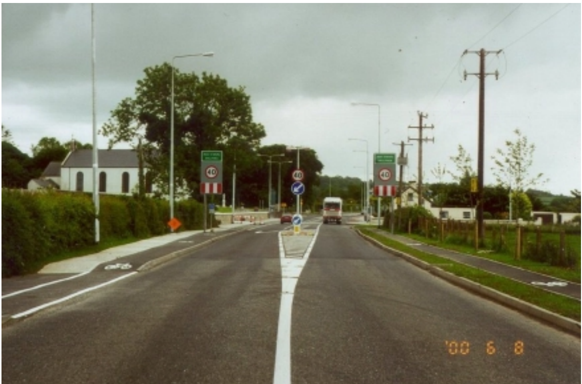
Photo 3: N20 Ballyhea, Co. Cork – North Approach ‘after’
