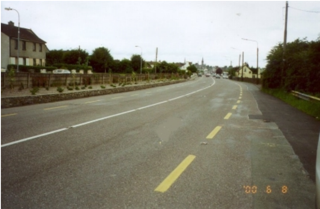
Photo 5: N20 Charleville (South), Co. Cork – Inside Gateway ‘before’
