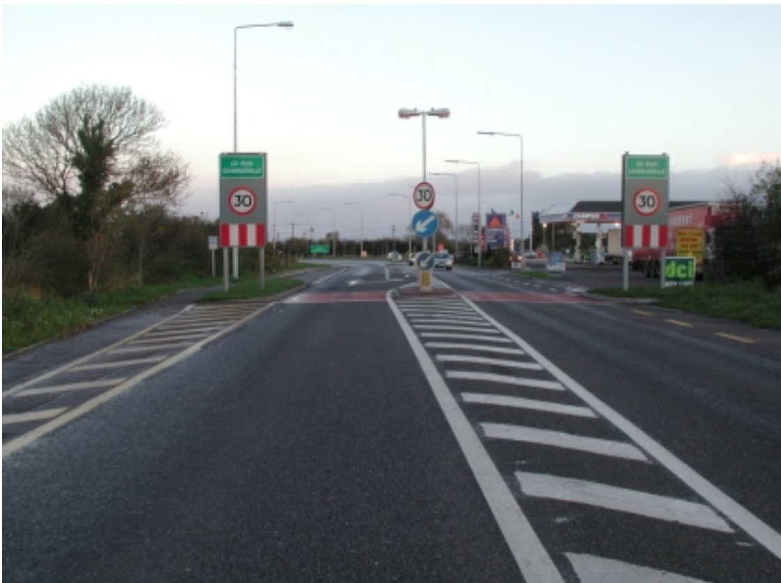
Photo 2: N20 Charleville (South), Co. Cork – South Approach ‘after’
