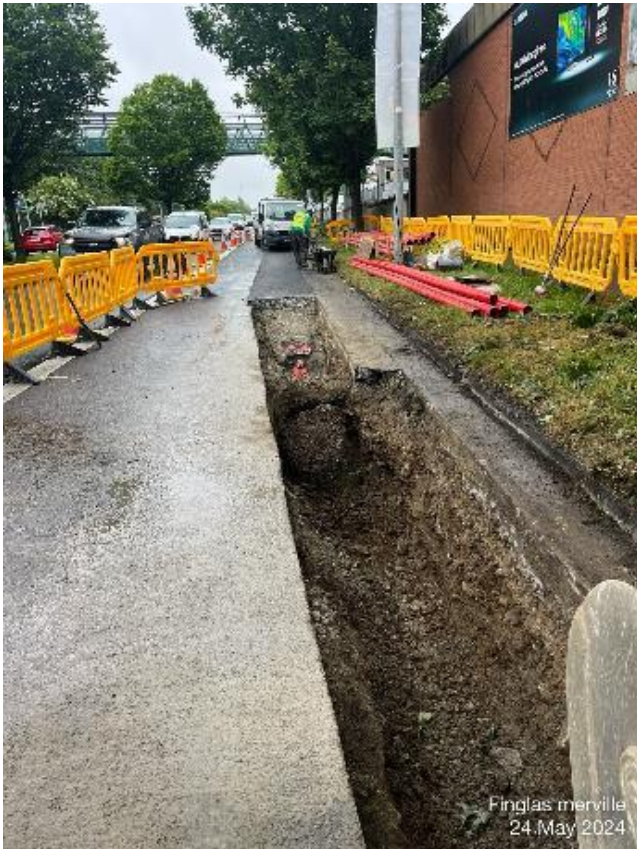
TM in place, road opened up
