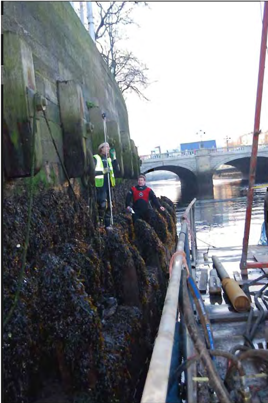
Plate 29: West-facing view along Burgh Quay showing total station recording of the timber revetment; plate annotated to show Type G timbers.
