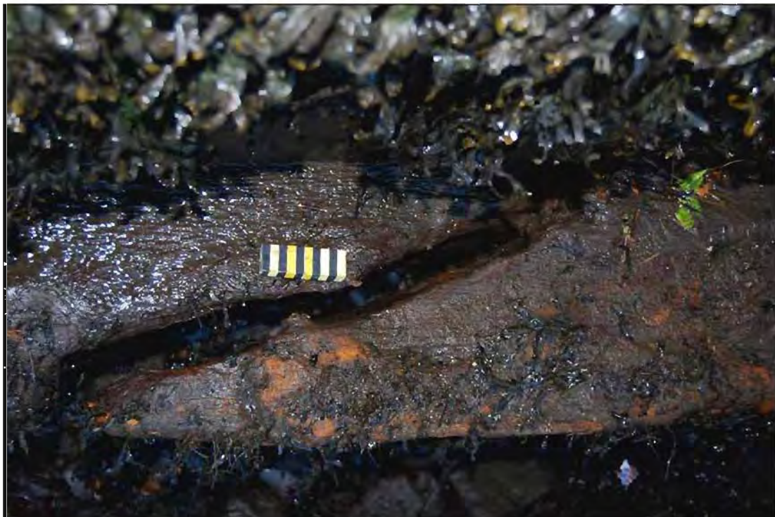
Plate 25: Detail shot of vertical Scarph-joint used to fasten the horizontal timbers (Type D) that run along Burgh Quay (Feature 2); 0.10m scale.
