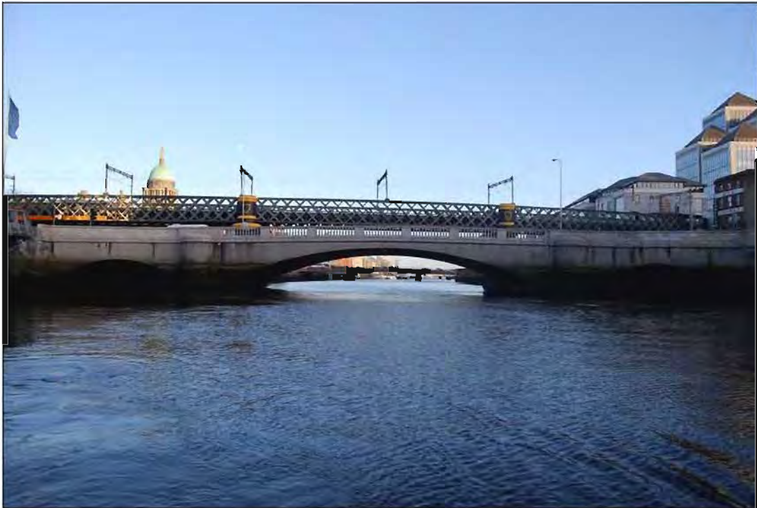
Plate 11: East-facing view of upstream façade of Butt Bridge.
