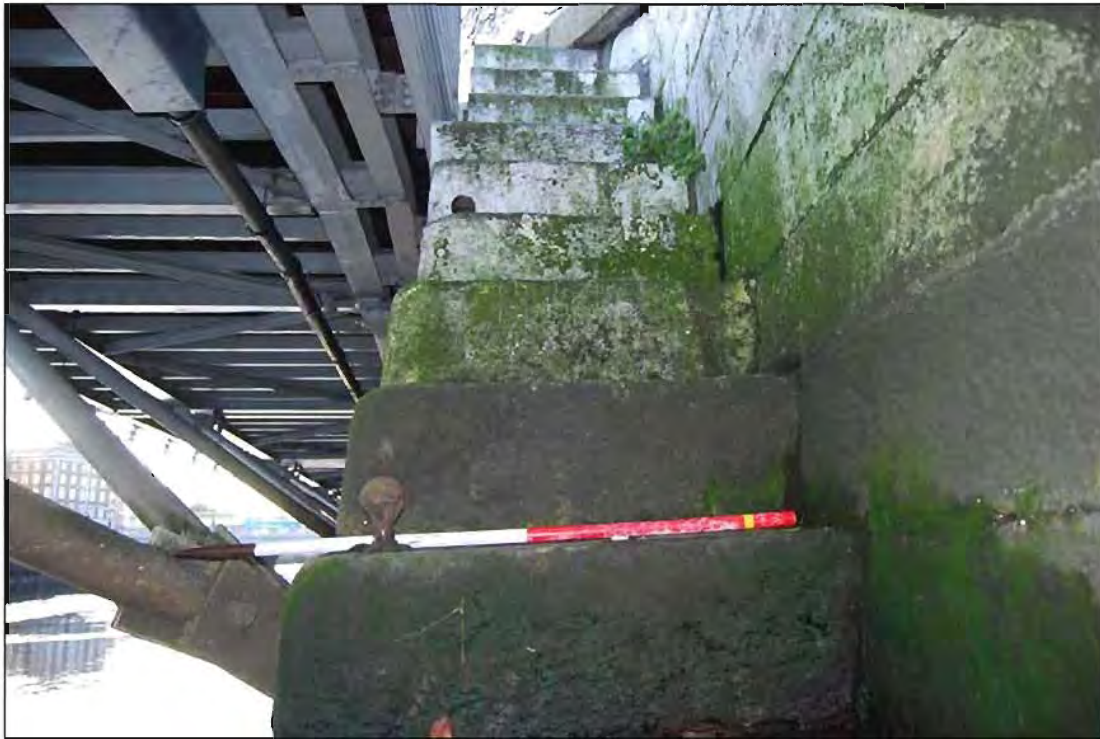
Plate 32: East-facing detail shot of masonry steps providing access to the river from Eden Quay (Feature 3); 1m scale.
