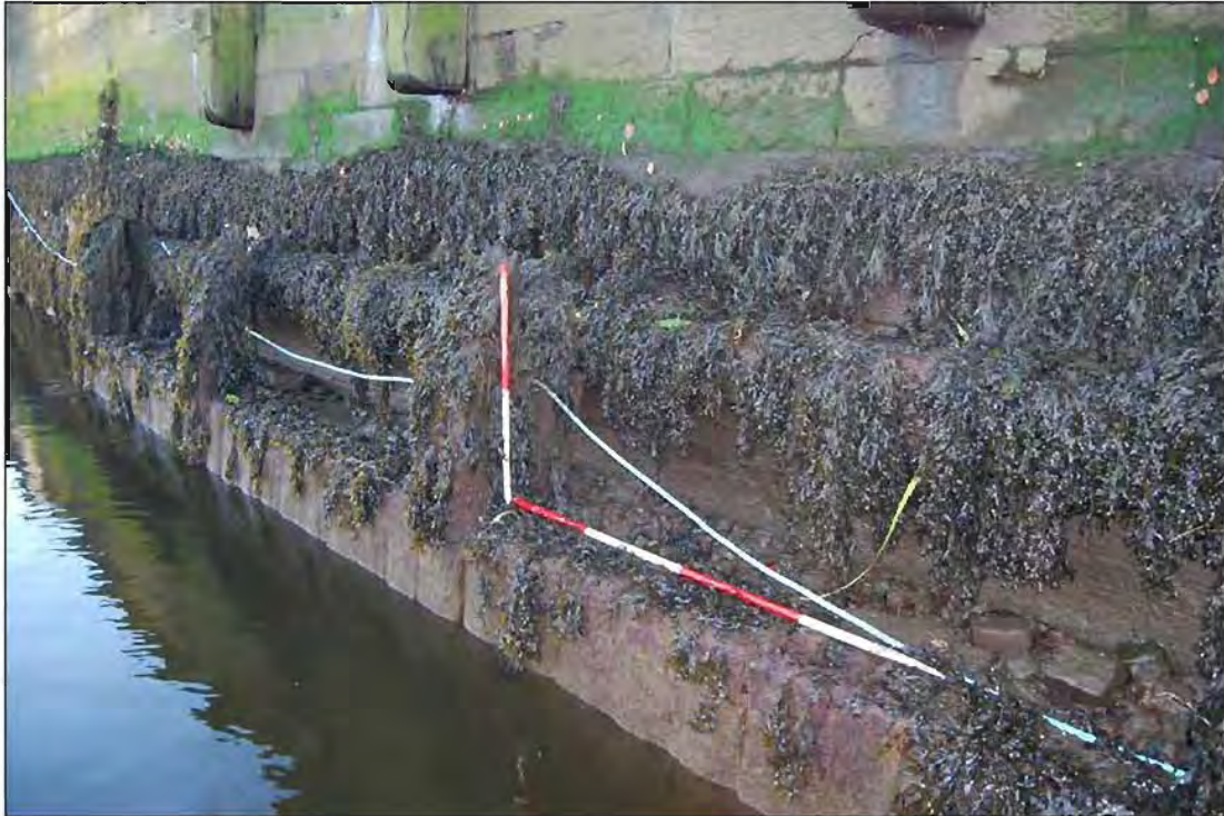
Plate 24: Detail shot of timber revetment at Burgh Quay (Feature 2) showing vertical Timber Types A, B, and C; horizontal scale 2m, vertical scale 1m.
