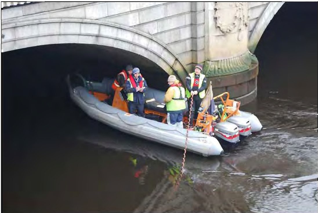
Plate 15: Working shot of dive set-up during underwater survey undertaken along the downstream side of O'Connell Bridge.
