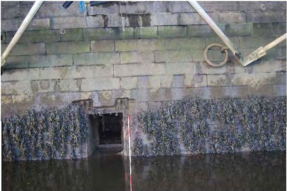
Plate 31: North-facing view of nineteenth-century drain located along the base of Eden Quay (Feature 3); 1m scale.
