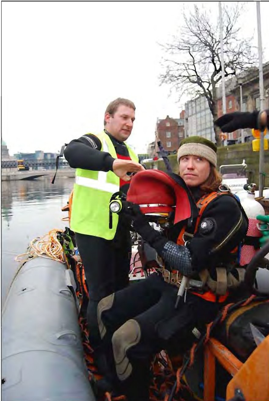
Plate 13: Working shot showing diver preparing for water. Note: diver using mobile Surface-supplied diving set-up.
