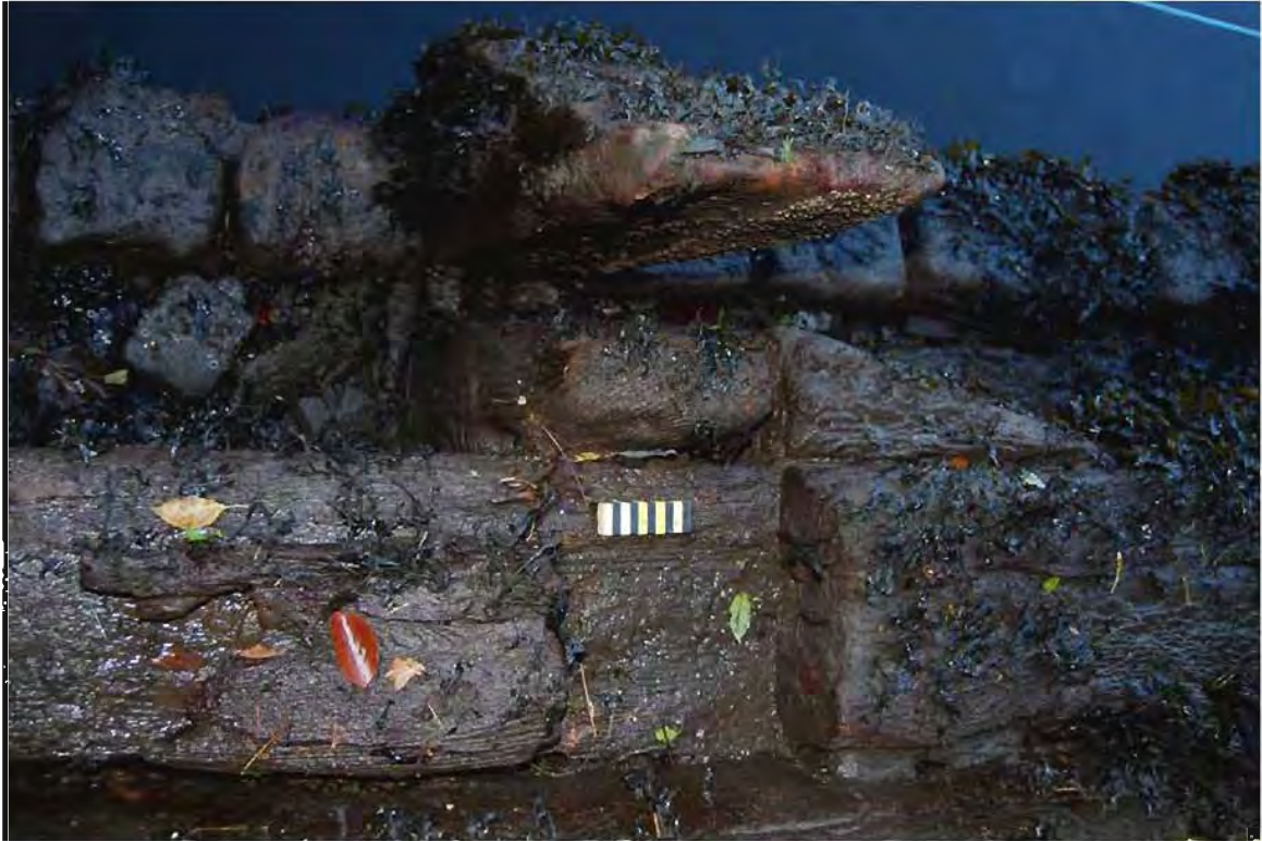
Plate 26: Plan view of composite section of timber revetment at Burgh Quay (Feature 2) showing timber types A, B, C, D, and the wedge-shape timber type E.; 0.10m scale.
