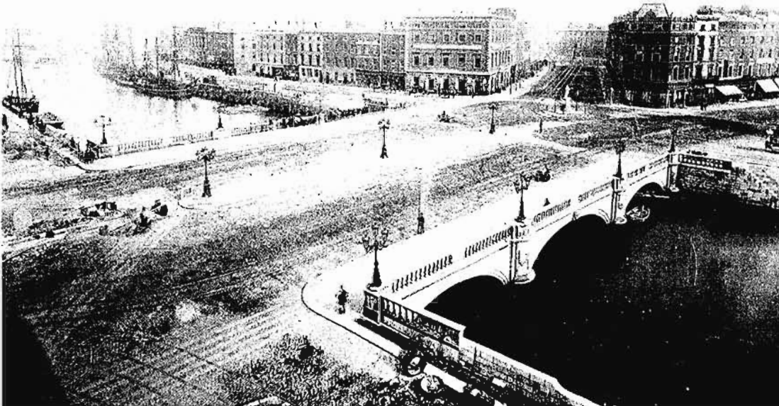
Plate 8: Photograph of O'Connell Bridge near completion in 1880; note shipping moored along Burgh Quay and Astor Quay.
