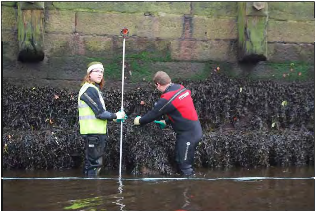
Plate 12: Working shot of Total Station survey of the Timber Revetment located alongside Burgh Quay (Feature 2).
