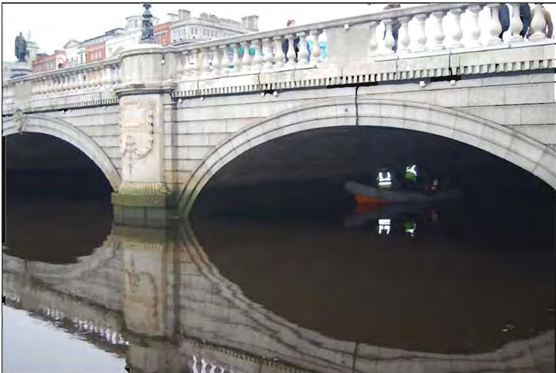
Plate 17: Working shot of diver preparing to enter water at start of underwater survey of the southern arch of O'Connell Bridge.
