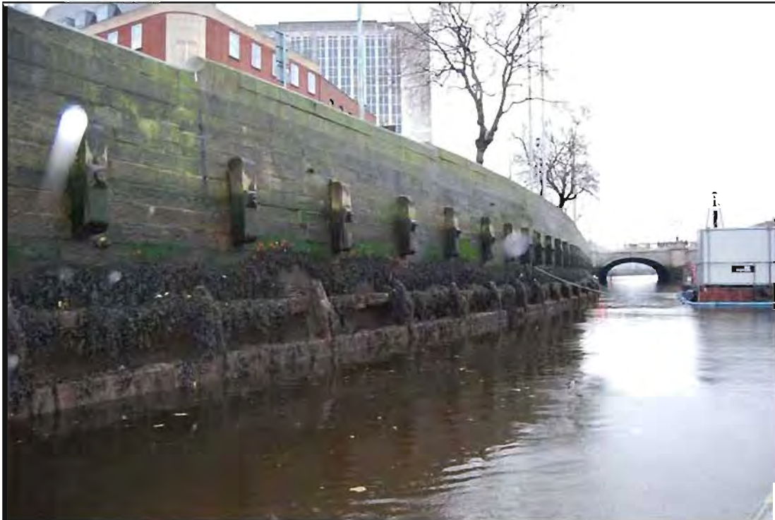
Plate 22: Southwest-facing view along Burgh Quay (Feature 2) and its associated timber revetment; O'Connell Bridge in distance.
