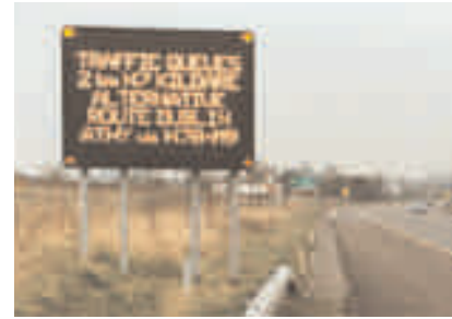
Example of a VMS Display
