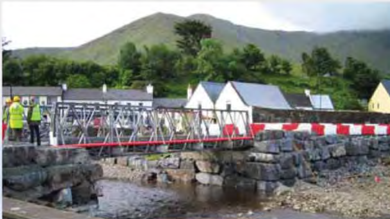
N59 Bridge Replacement, Lennane (before)
