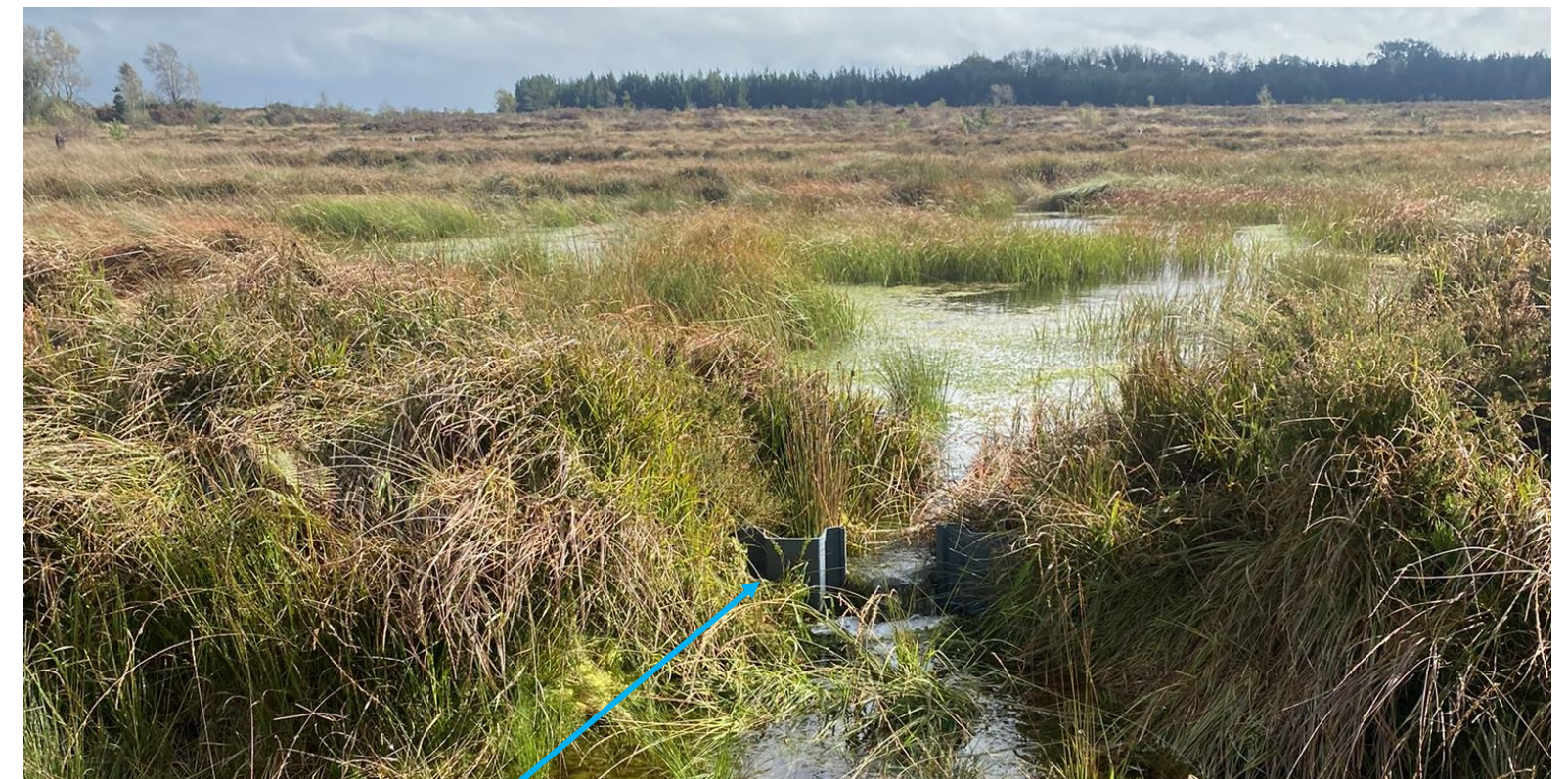
Drain blocking for peatland restoration
