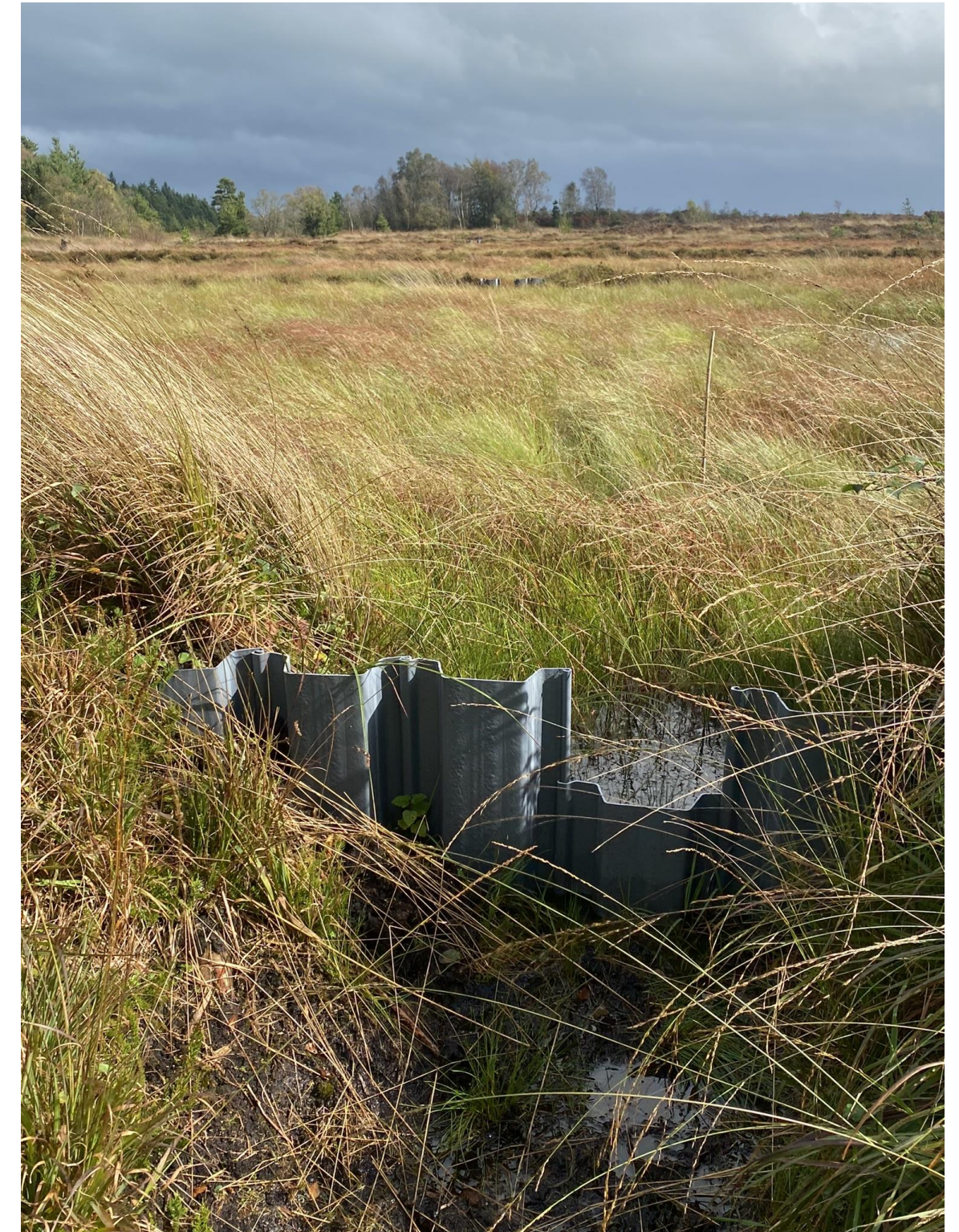
Peat Drain Dam (Plastic Sheet Piles) at Cloncroe Bog
