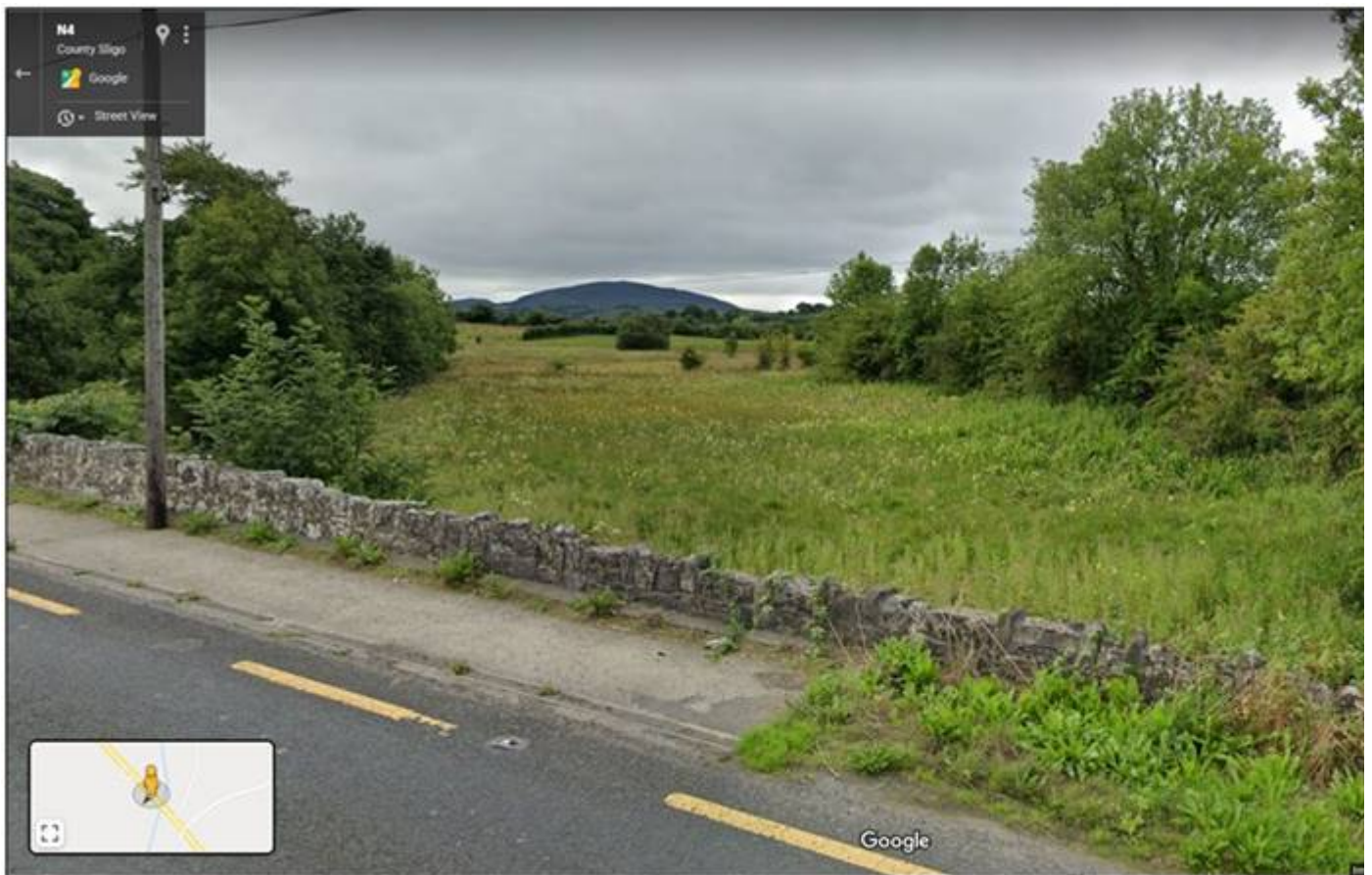
Upstream of Behy Bridge (Source: Google Street view Aug 2018) ( https://goo.gl/maps/ZEUppsSoE8rxS6vg9 ).
