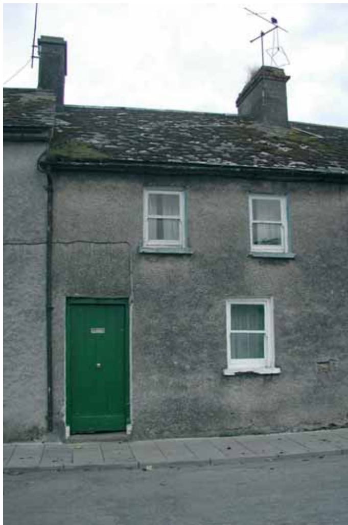
Figure 5 Vernacular buildings may also have heritage merit
