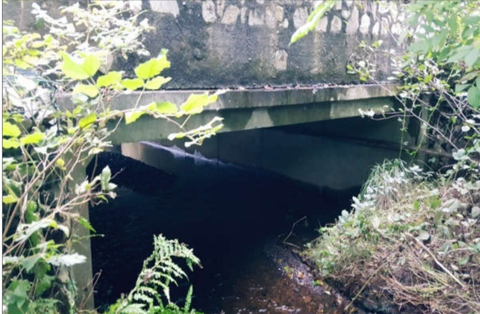
Plate 2-6 N56 Barnes Bridge.
