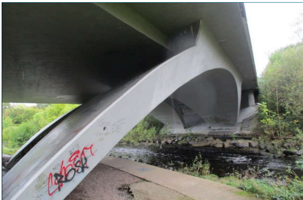
Plate 5-2 River Eske Bridge.
