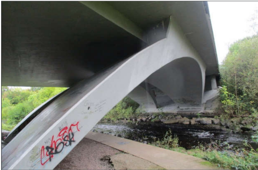
Plate 2-2 River Eske Bridge.
