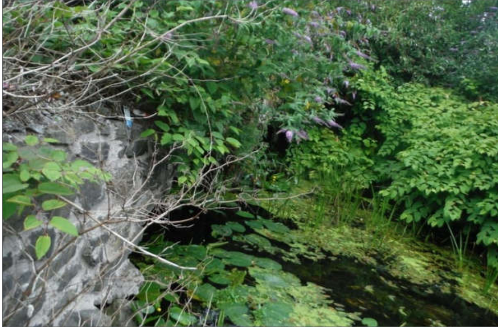
Plate 2-8 Terryland River Bridge No. 3.
