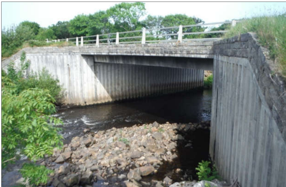
Plate 2-12 Banduff River Bridge.
