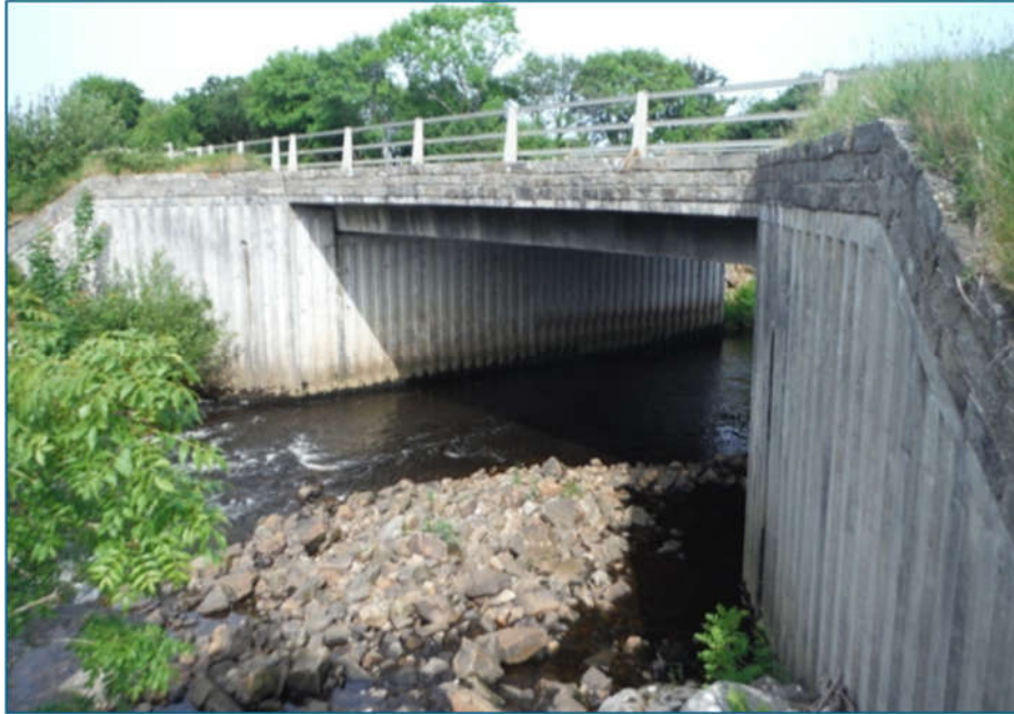
Plate 5-12 Bunduff River Bridge.
