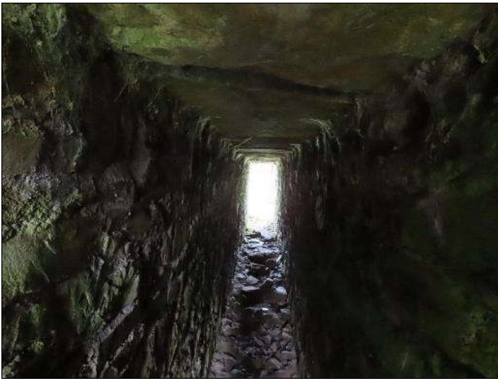
Plate 4.6 View under centre clapper.
