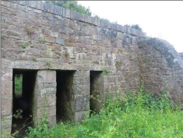
Plate 4.27 Upstream face of Western Flood Pass.
