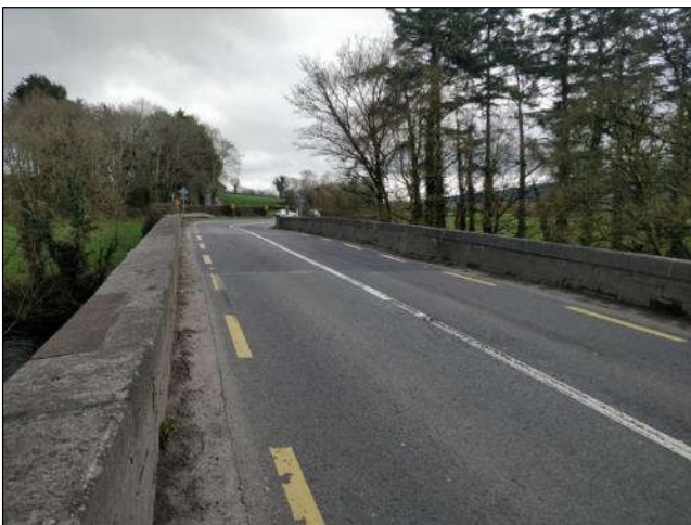
Plate 1.9 View of road above Leader's Bridge.
