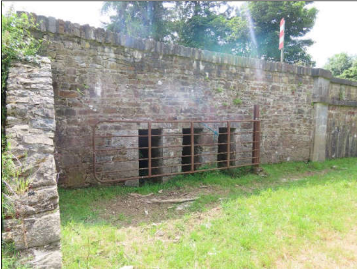
Plate 4.8 Upstream elevation showing stonework in good structural repair.
