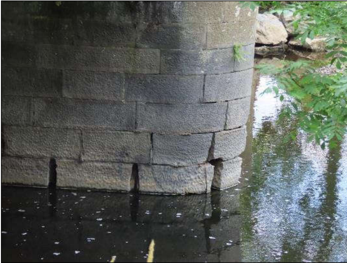
Plate 4.11 Close-up of base of abutment and upstream pier of easternmost arch.
