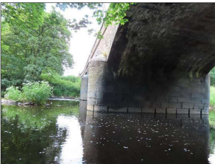
Plate 4.13 Stonework at base of abutment of centre arch.
