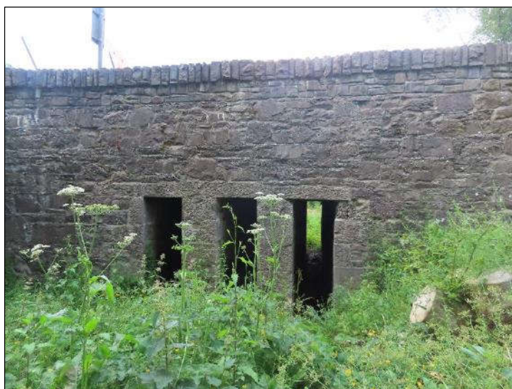
Plate 4.26 Downstream face of western flood pass.
