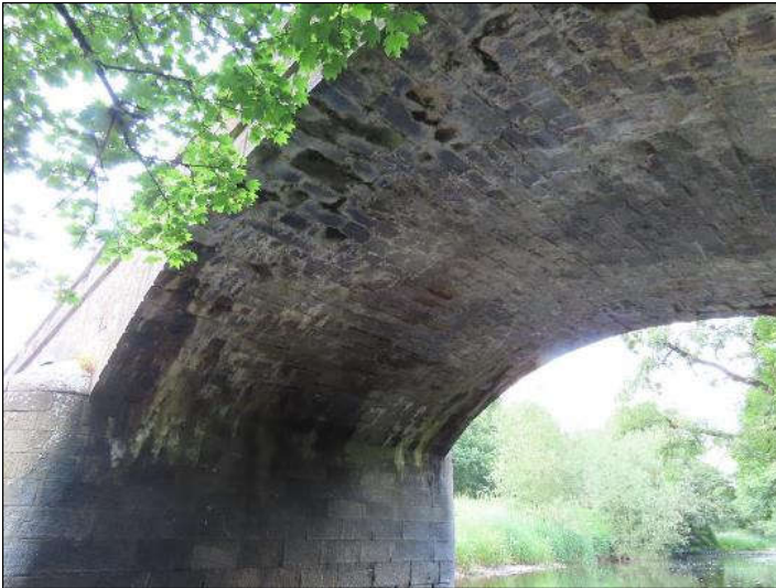
Plate 4.12 Under surface of easternmost arch – no crevices between stones.
