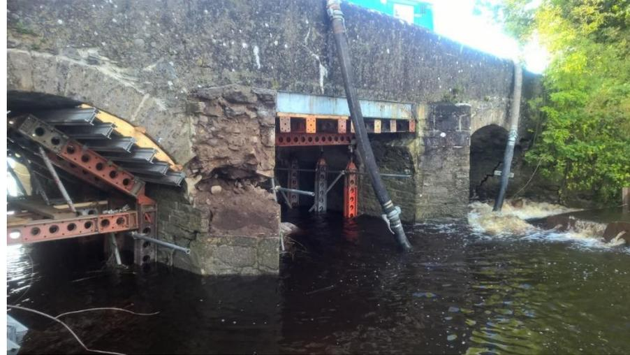
Bridges with shallow foundations are most susceptible to scour damage from erosion of the river bed
