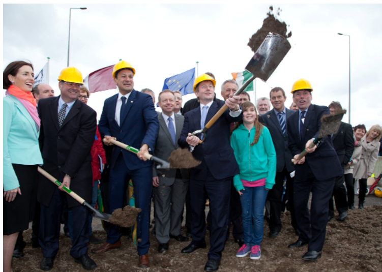
The sod turning of the M17/M18 Gort to Tuam Motorway
