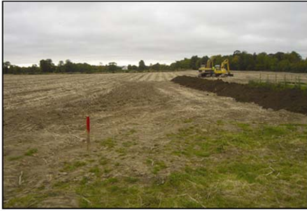
Plate 1 - Test area 5 sub area 12, general pre-excitation.
