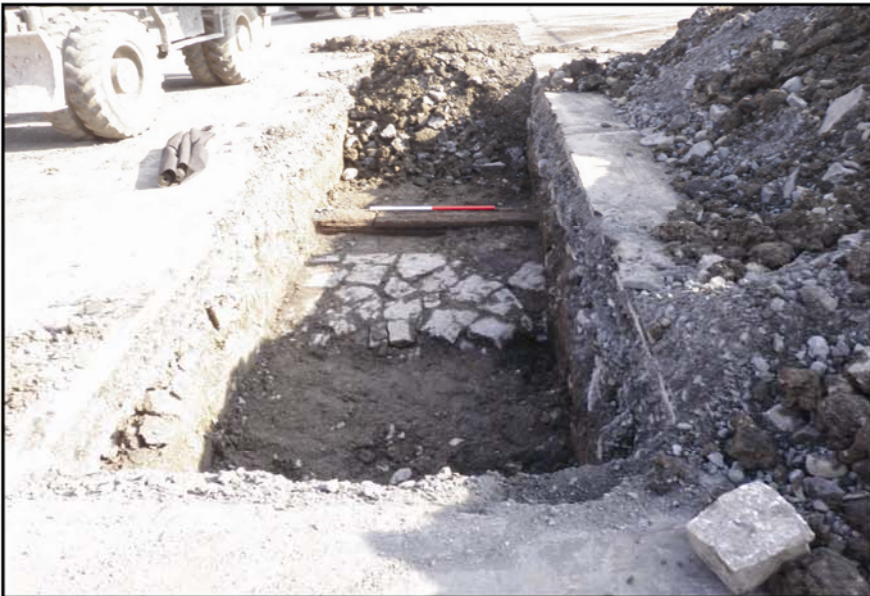
Plate 11 - Mid-excavation of Trench 2, showing possible slipway, southeast facing
