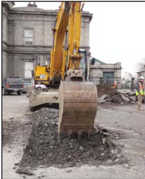
Plate 7 - Mid-excavation of asphalt removal Trench 2, northwest facing
