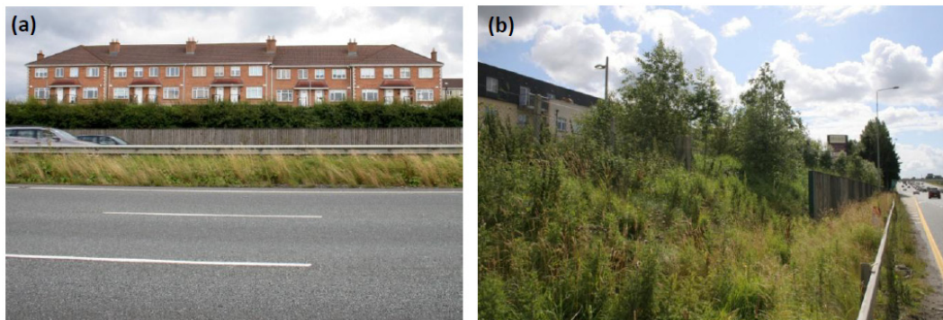
Figure B.4 - Noise Barrier installations where line of sight is not blocked
