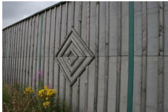
Figure B.17 -Absorptive barriers with vertical battens helping to break up monotony
