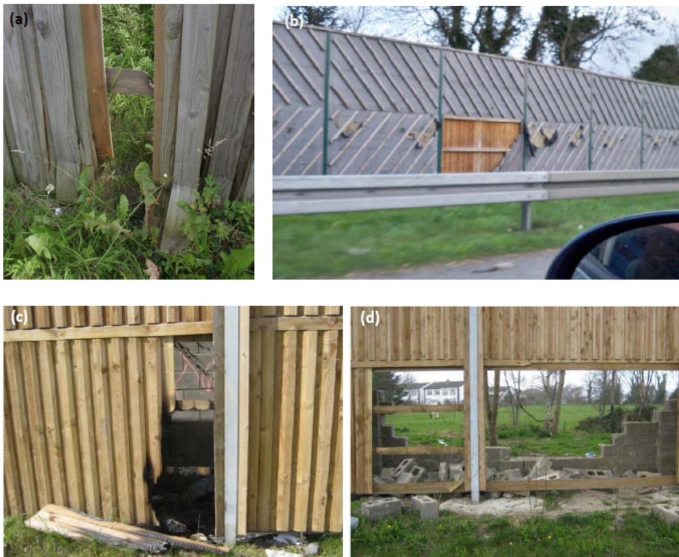
Figure B.23 - Examples of damage to timber noise barriers due to vandalism
