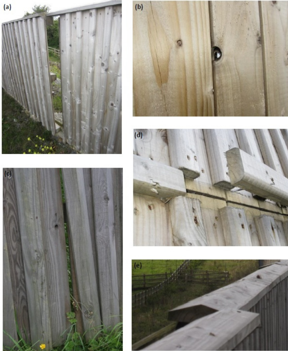
Figure B.21 - Damage/degraded protective membranes on absorptive noise barrier
