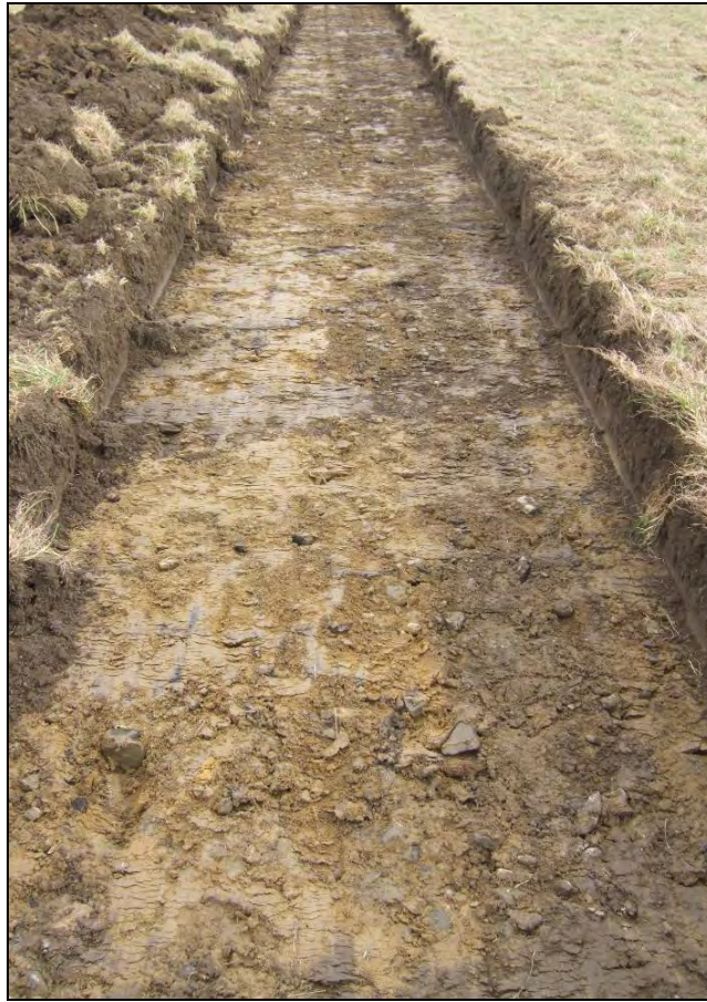
Plate 15: Drain C57 in TT 2 (TA A3), facing east
