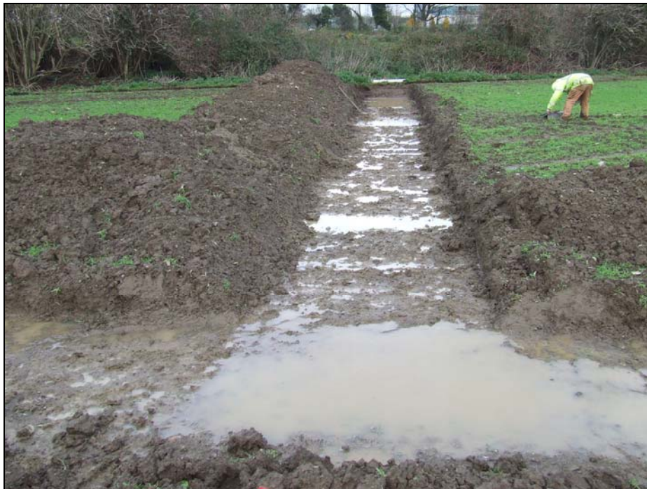
Plate 1: TT 1, facing north
