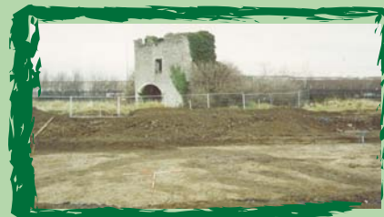
Site clearance at Ballymount
