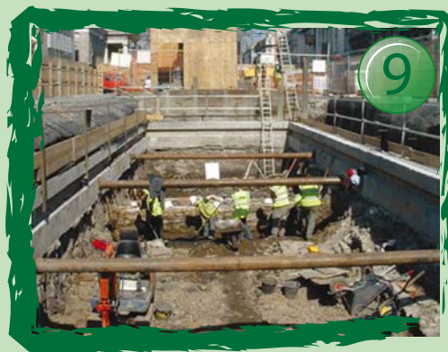
Work at O'Connell Street
