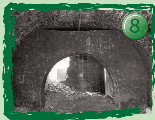
Vault 14 at Connolly Station
