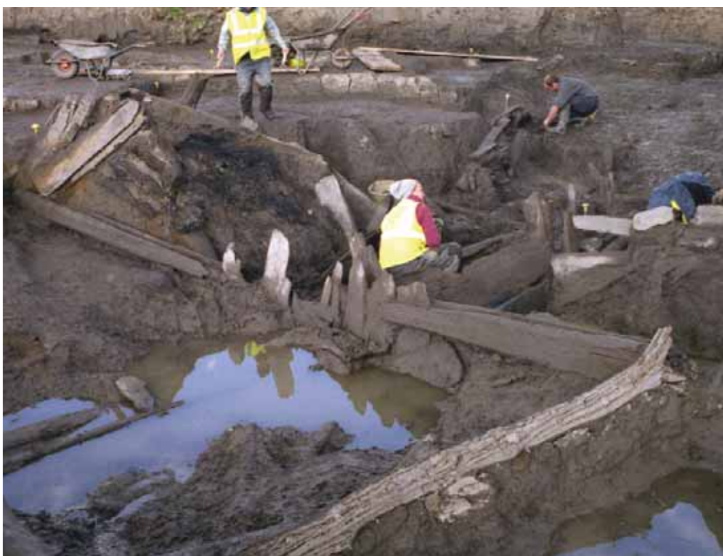
Illus. 5—Photograph of wheel-pit under excavation, showing rectangular opening in lower dam (Archaeological Consultancy Services Ltd)
